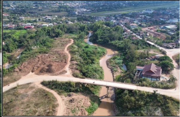
Nam Kor Bridge 4
