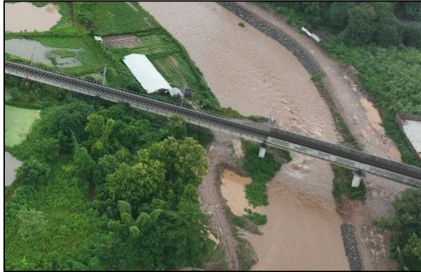
Railway Bridge at the Nam Mao River
