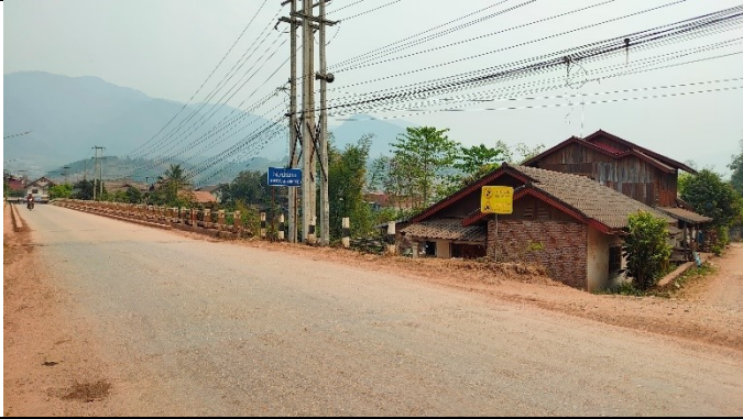
Installation of warning signs at 0+000 L in Nasao Village
