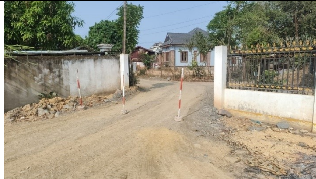
Site barricades with gate at km 1+900 L Pasak village
