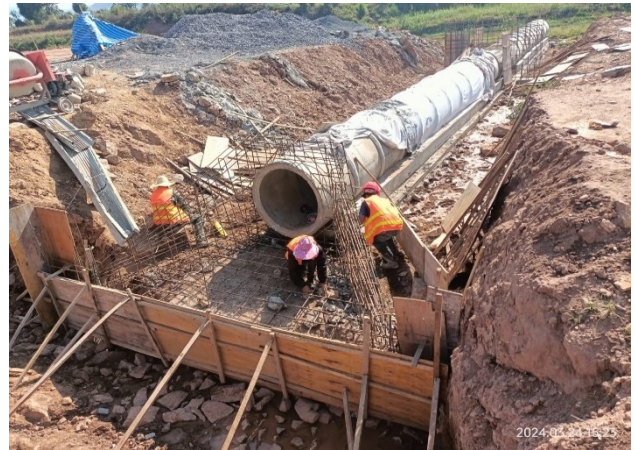
Existing conditions of Drainage/Gate
