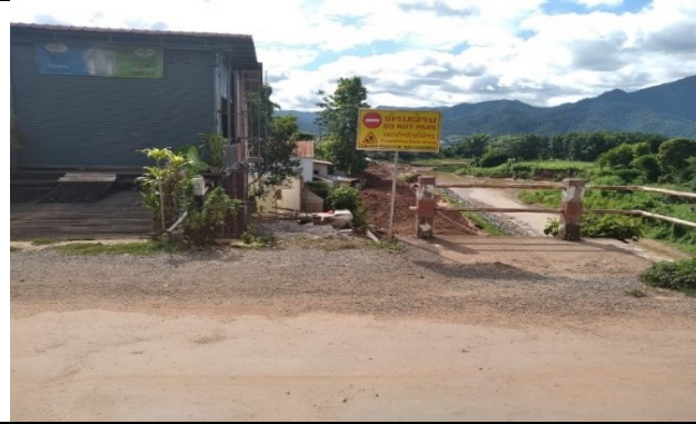
Installation of warning signs at 0+350 L in Thin village
