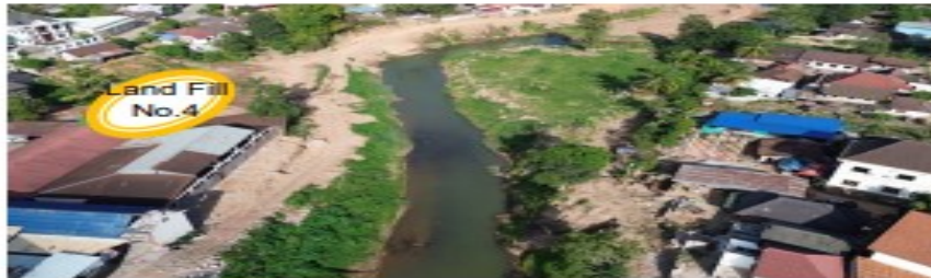
Land fill No.4 Section L-2 Km 1+210 to 1+275
