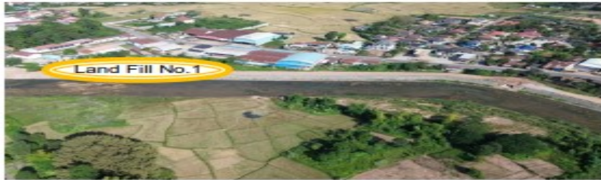
Land fill No.1 Section R-1 Km 1+500 to 1+600
