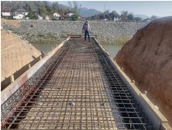
Existing conditions of Drainage/Gate
