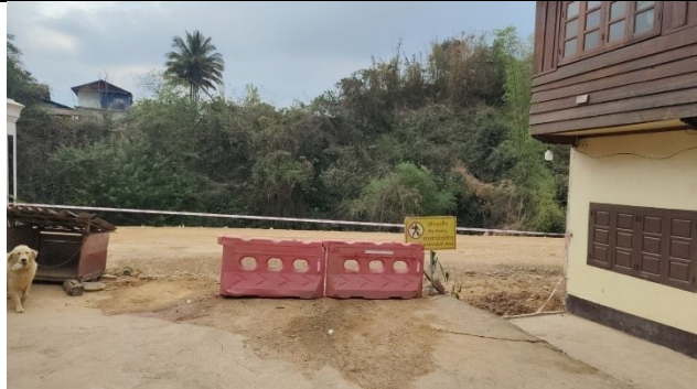
Site barricades with gate at km 1+900 L Pasak village
