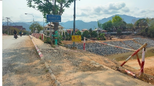
Installation of site barricades (red-and-white vinyl tape) and warning signs at the construction site
