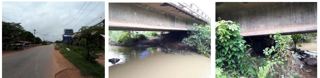
Bridge No.02 Houay Xai Moun at Km 7+019
