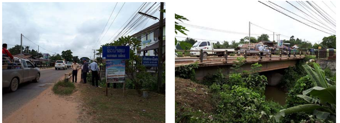
Bridge No.03 Nam Houm at Km 19+250
