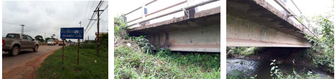
Bridge No.01 Houay Xon at Km 10+053
