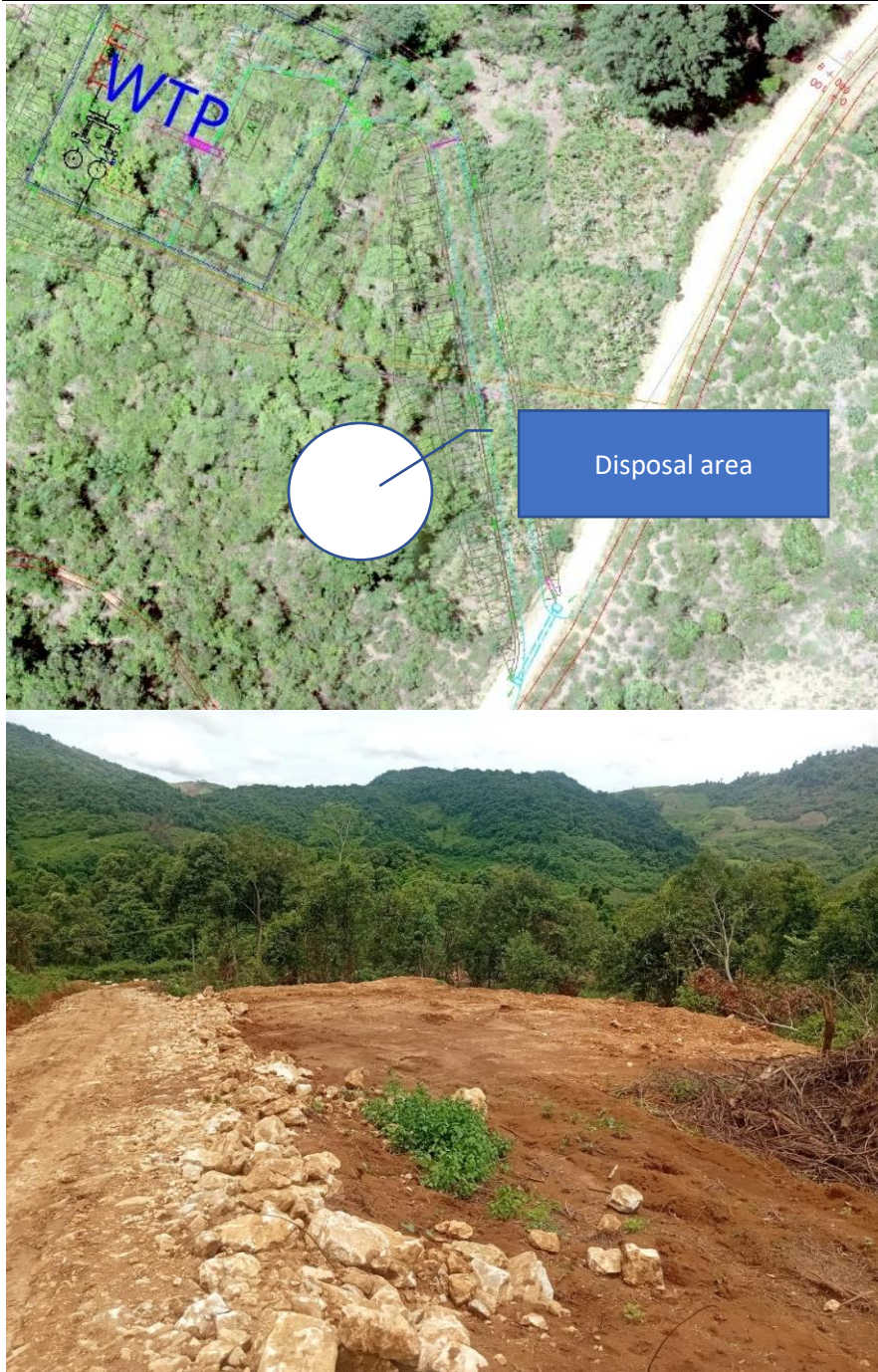
FIGURE 5-5 PROPOSED OF THE SPOIL DISPOSAL SITES FOR WSS MUANGNA CLUSTER IN KOUAN DISTRICT
