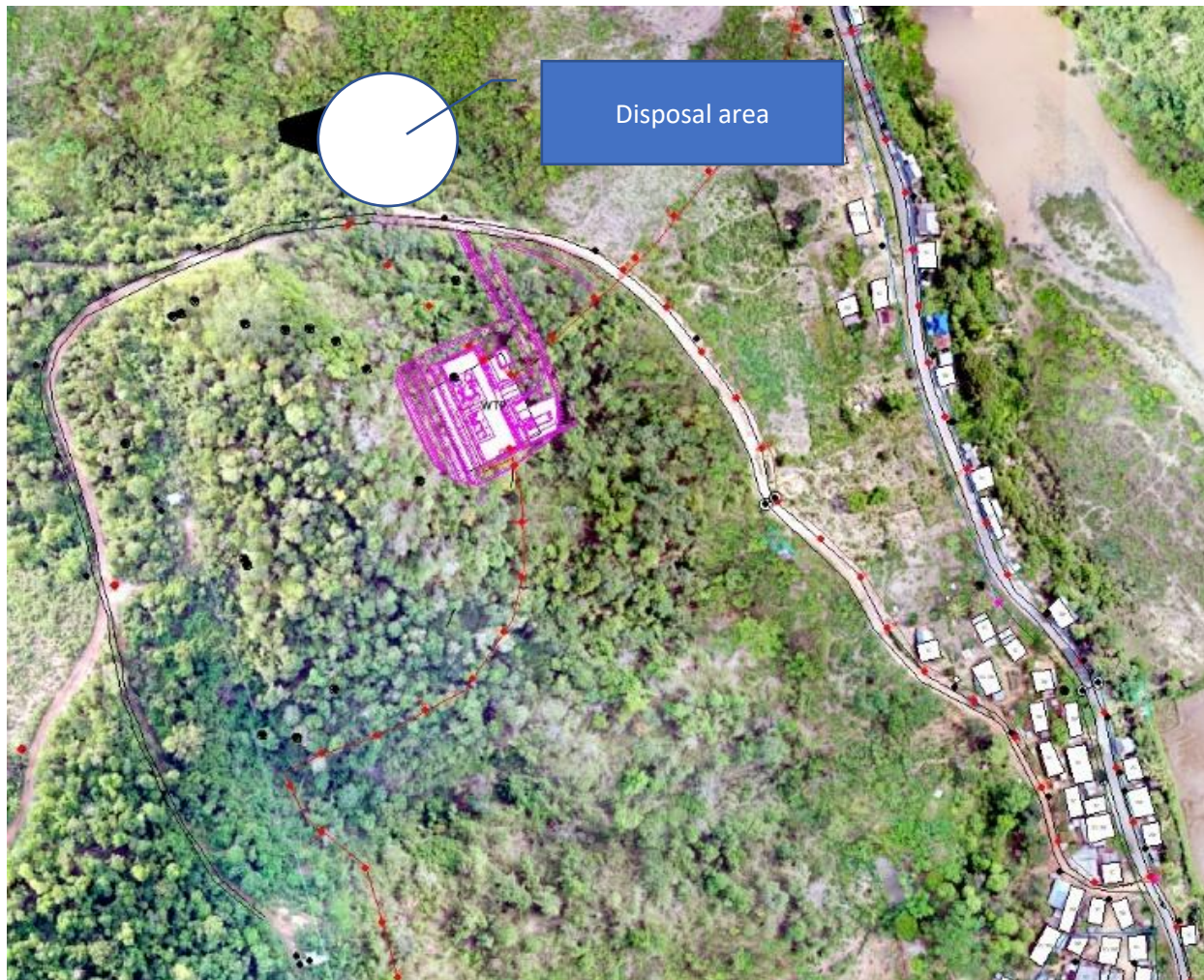
FIGURE 5-6 PROPOSED OF THE SPOIL DISPOSAL SITES FOR WSS PHANXAM CLUSTER IN XAMTAY DISTRICT
