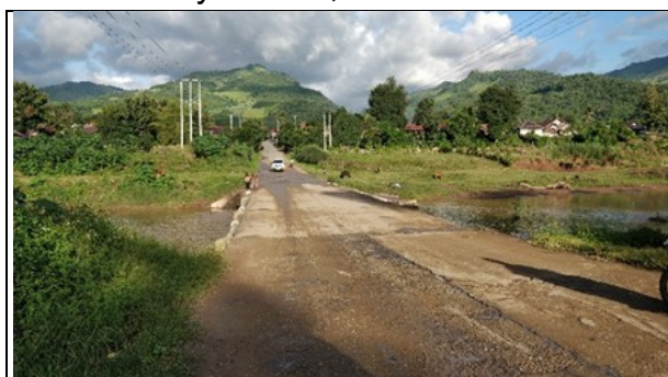
Plate 3-1 Water crossing along NR2 West
