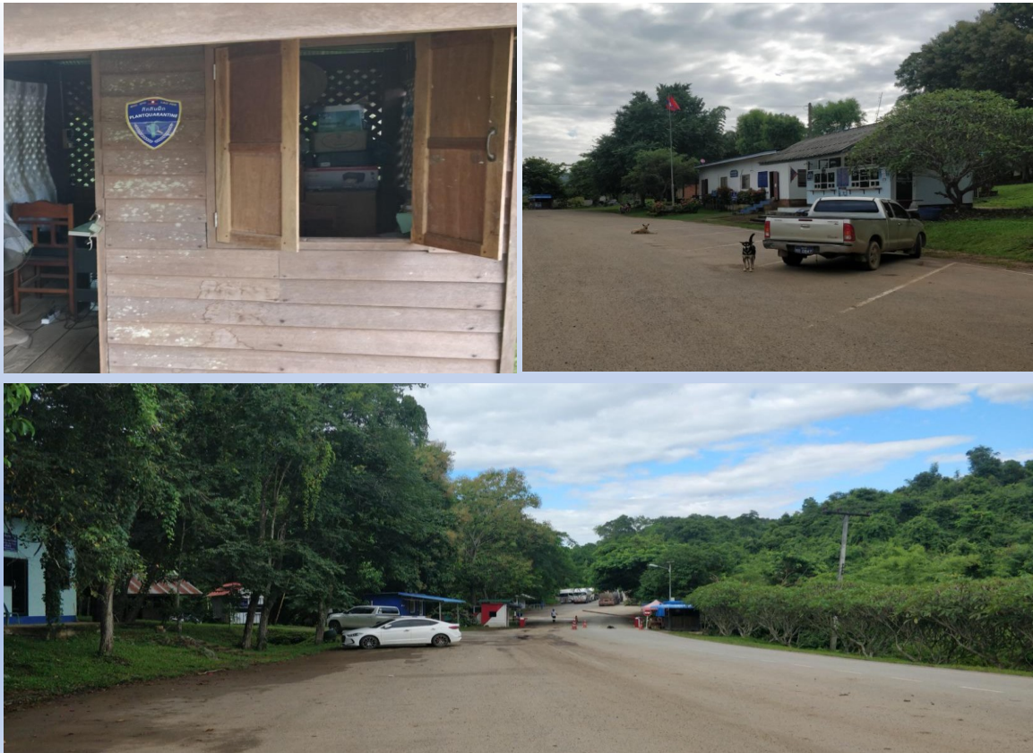
Photo 5: Existing Structures in the Nam Ngeun BCF
