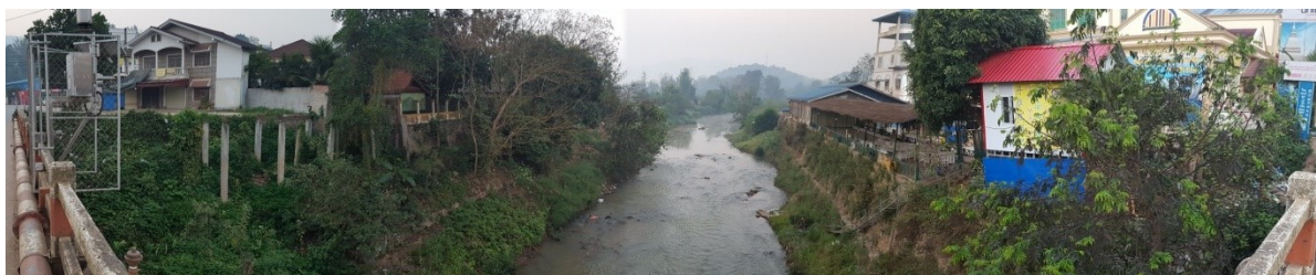
Figure A3-4 Present Condition at the Downstream of Nam Kor Bridge 5
