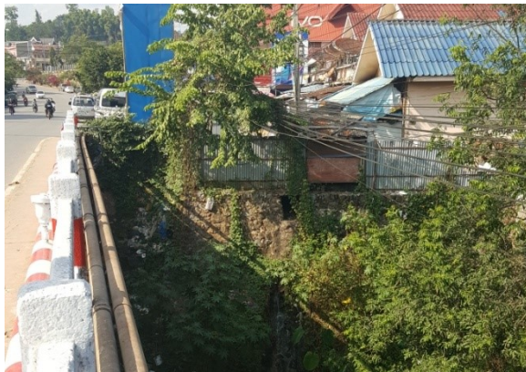
Drainage Outlet near the Market
