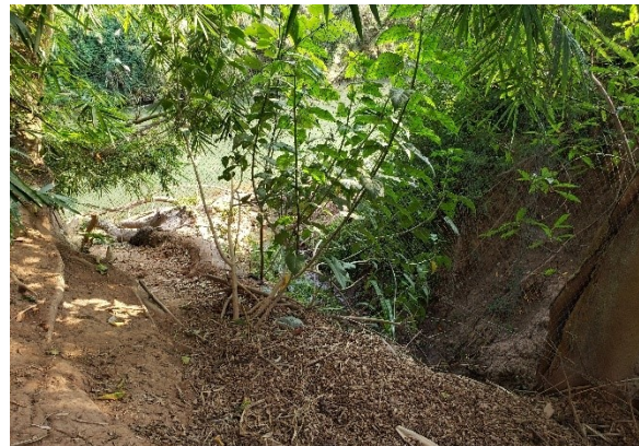
Drainage Outlet near the Stadium
