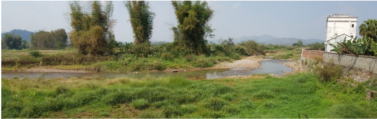
Figure A3-5 Present Condition at the Downstream of the Nam Mao Bridge
