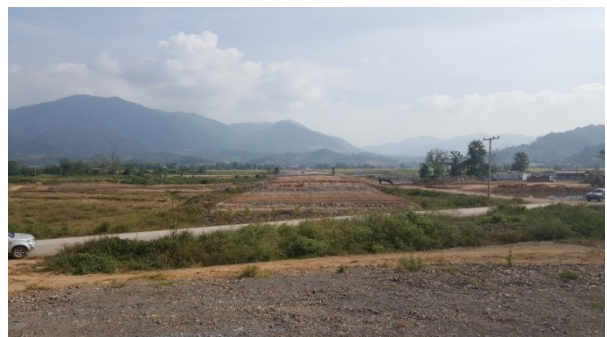
Rapid Railway under Construction
