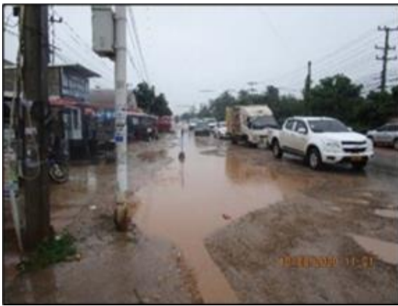
No existing ditch (pavement edges are severely deteriorated)
