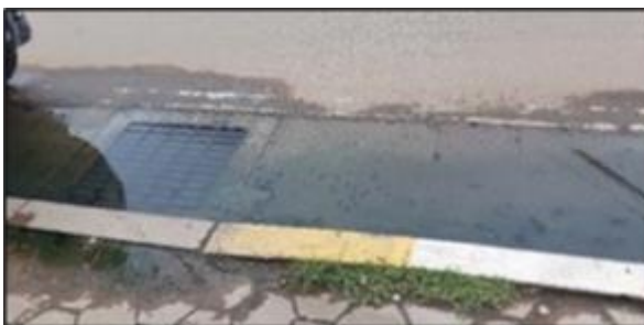
Existing Gully and Manhole (in the area of start point there is lack of maintenance, full of debris and sediment)
