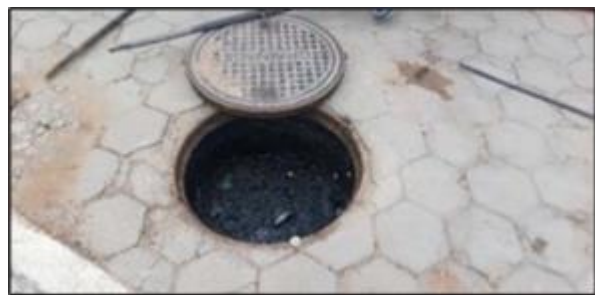
Existing Gully and Manhole (in the area of start point there is lack of maintenance, full of debris and sediment)
