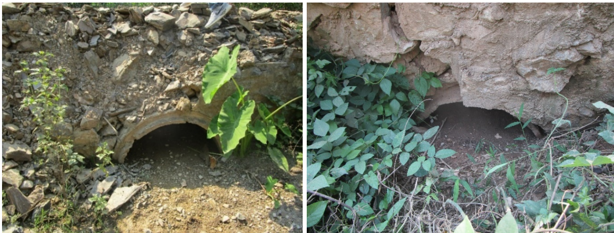
Figure 3. Pipe culvert on Km 15+120 and Km 15+590, Local Road No. 2571
