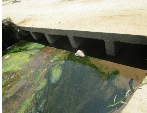
Figure 4. Submersible Bridge (Km 7+980), Local Road No. 2571
