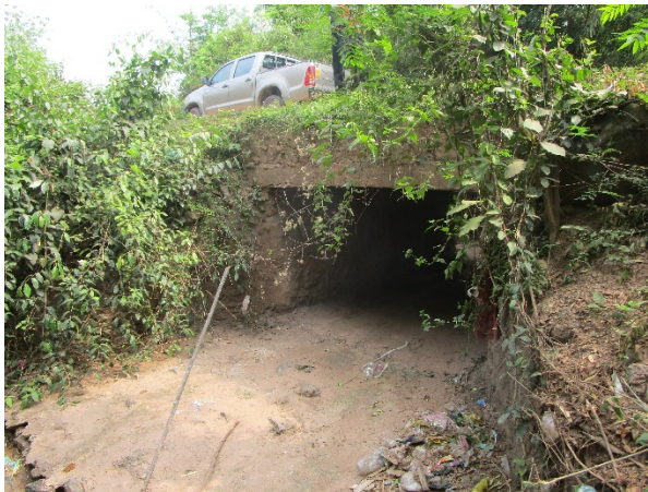
Figure 11. Box culvert on Km 2+700 and Km 8+100, Local Road No. 2652
