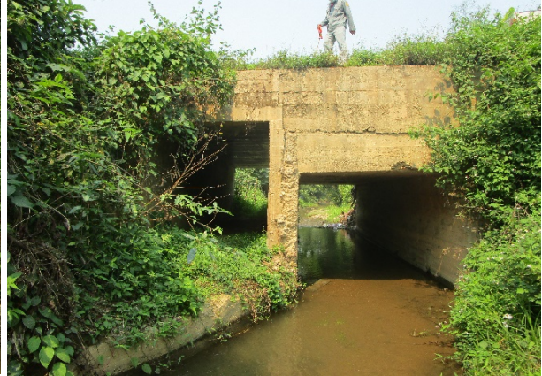
Figure 22. Pipe culvert (Km 2+610) and Box culvert (Km 5+750), Local Road No. 2931-3170
