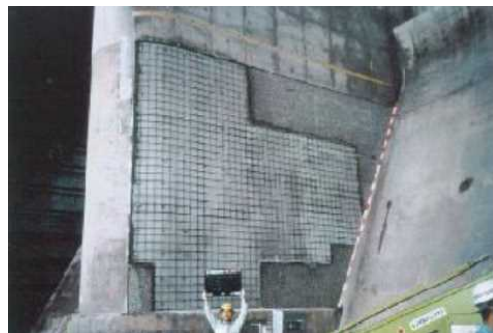
Cleaning of Concrete and Rebar
