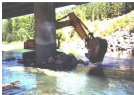
Figure AP 1.13.4 Placing Rip Rap
