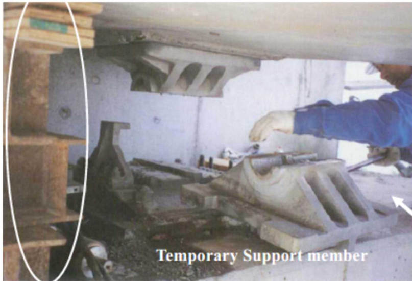
Sample of Replacement Bearing by Jack-up Girder
