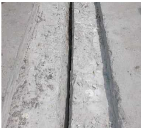
Cleaning of the gap
