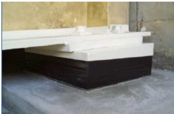
Sample of Replacement Bearing
