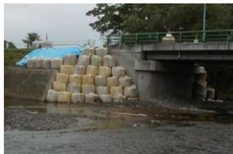
Figure AP 1.13.3 Placing Sand Bags
