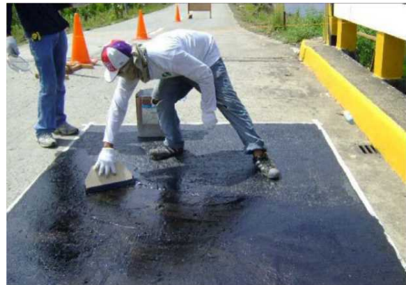
Figure AP 1.10.2 Asphalt Compound Membrane Type
