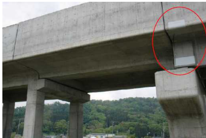
Figure AP1.6.1 Protective Coating applied on Surface of Superstructure
