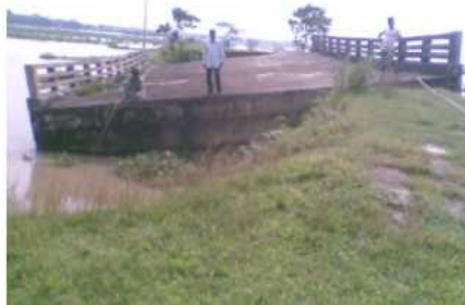
Figure AP 1.13.1 Typical Bridge Scour
