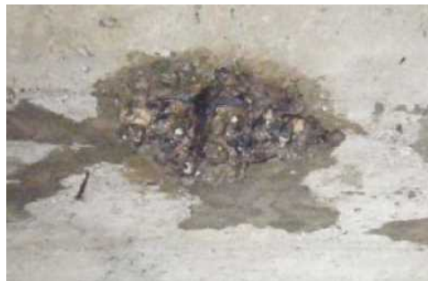
Epoxy Bonding Coat
