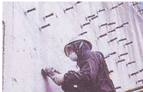
Figure AP1.1.2 Injection of repair material
