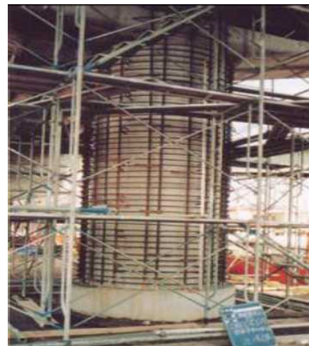
Figure AP 2.7.2 Concrete Wrapping for Repair Pier
