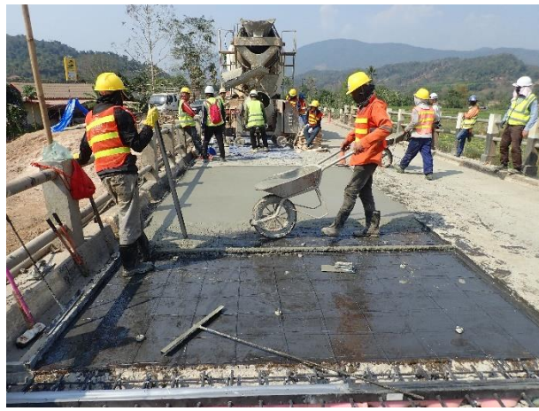
Compact Jet Concrete casting on Bridge Surface Span 1 - Span 2 L/S on 24 th February 2023. (SP 1 – SP 2 L/S: W= 3.25m, L= 17.90m)
