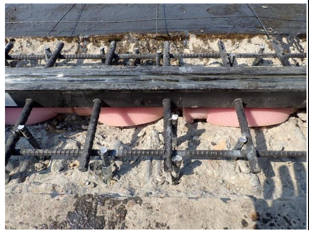
Installation of Expansion Joint (L= 3.46 m) at P1 L/S on 24 th February 2023.
