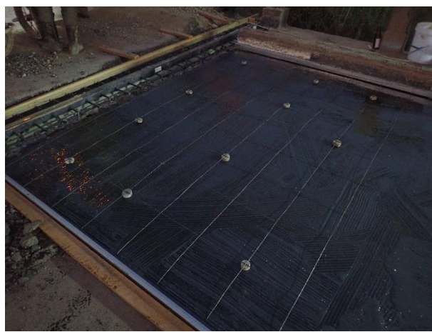
Set up the Wire mesh and Compact Jet Concrete casting on Bridge Surface Span-2 R/S on 20 th February 2023. (W= 2.70m, L= 20.0m)
