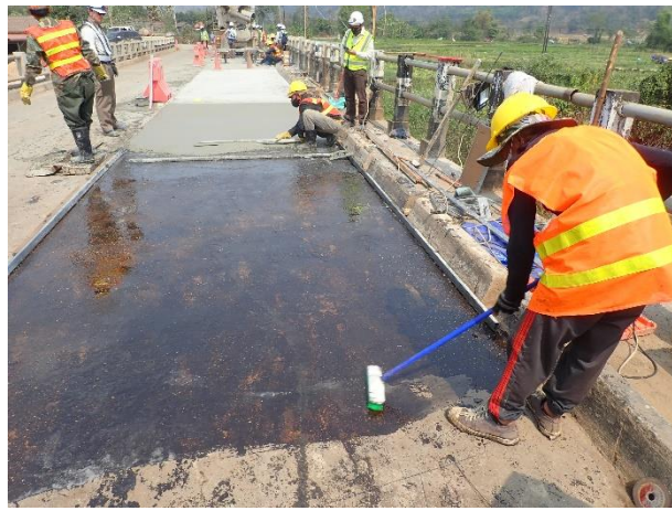
Application of Primer cort and Bond on Bridge Surface Span 2 R/S on 22 nd February 2023. (W= 2.70m, L= 19.3 m)
