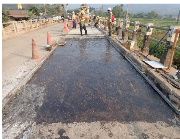
Application of Primer cort and Compact Jet Concrete casting on Bridge Surface Span1-2 R/S on 21 st February 2023. (W= 2.70m, L= 4.0m)
