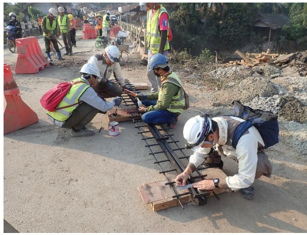
Installation of Expansion Joint at A1 R/S and A2 L/S on 22 nd February 2023.
