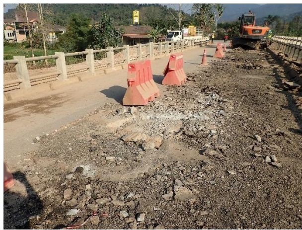
Removal of Existing pavement work on Bridge Surface Right side on 16 th February 2023
