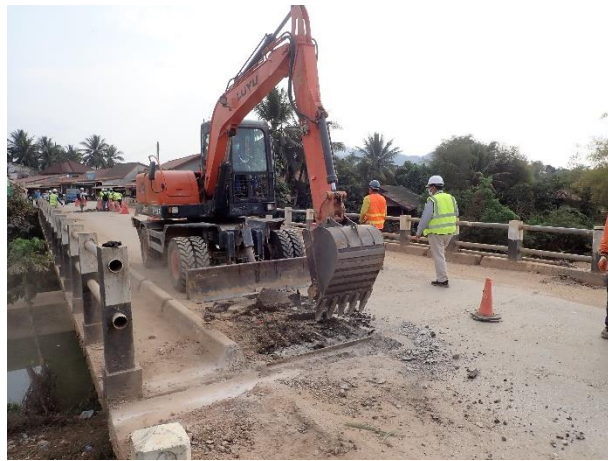
Removal of Existing pavement work on Bridge Surface Right side on 15 th February 2023
