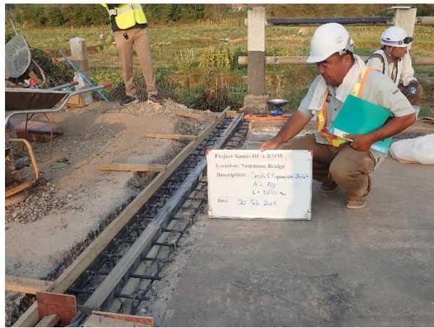
Installation of Expansion Joint (L= 3.65m) at A2 R/S on 20 th February 2023.
