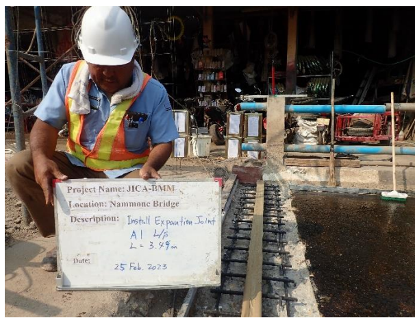
Installation of Expansion Joint (L= 3.49 m) at A1 L/S on 25 th February 2023.
