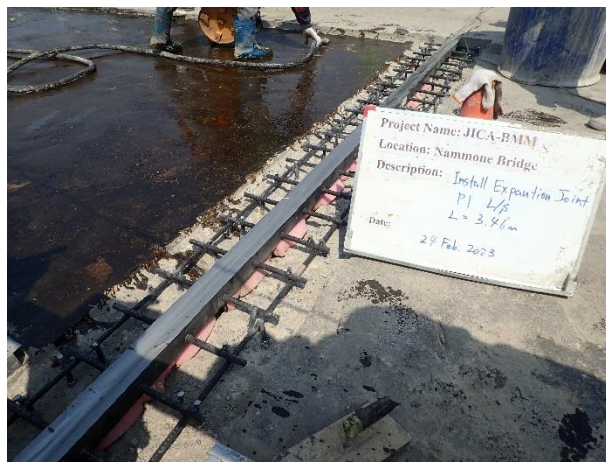
Installation of Expansion Joint (L= 3.46 m) at P1 L/S on 24 th February 2023.
