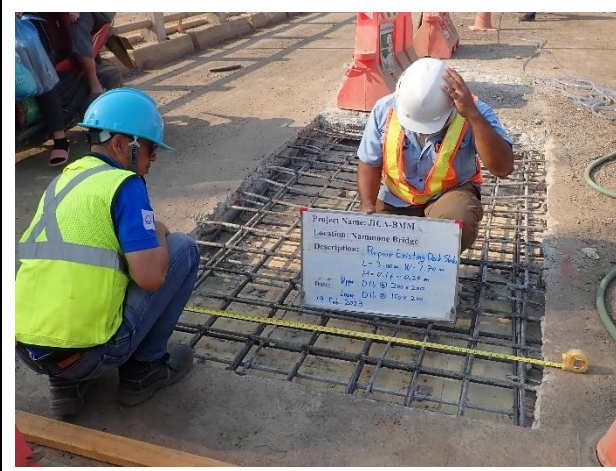
Inspection for Reinforcing bar and Formwork for the Expose area on Existing Deck Slab on 19 th February 2023. (L= 3.00m, W= 1.70m, H= 0.17 – 0.24m)
