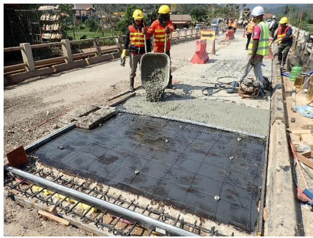
Compact Jet Concrete casting on Bridge Surface Span 1 R/S and Span 2 L/S on 23 rd February 2023. (SP 1 R/S: W= 2.70m, L= 3.5m, SP 2 L/S: W= 3.25m, L= 16.55m)
