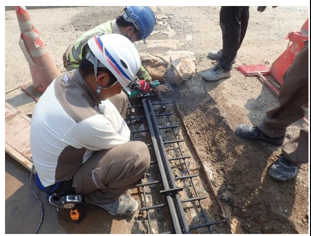
Installation of Expansion Joint at P1 L/S and A1 L/S on 24 th February 2023.
