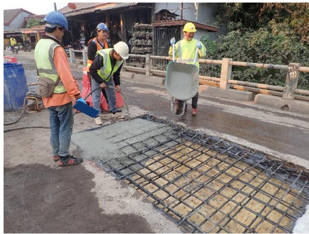
Concrete casting for for the Expose area on Existing Deck Slab on 20 th February 2023. (Trial Mix of Compact Jet Concrete; CPJ 1.05m 3 )
