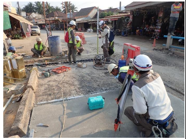
Installation of Expansion Joint at A1 R/S and A2 L/S on 22 nd February 2023.
