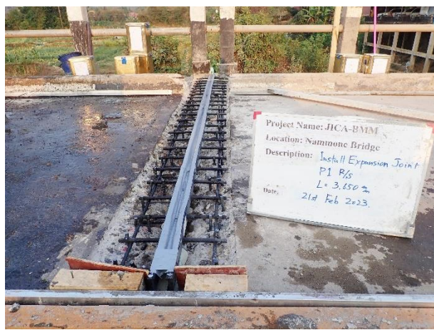
Installation of Expansion Joint (L= 3.65m) at P1 R/S on 21 st February 2023.
