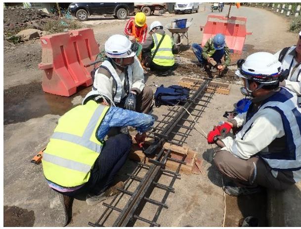
Installation of Expansion Joint (L= 3.65m) at A2 R/S on 19-20 th February 2023.
