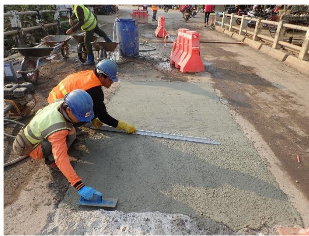
Concrete casting for for the Expose area on Existing Deck Slab on 20 th February 2023. (Trial Mix of Compact Jet Concrete; CPJ 1.05m 3 )
