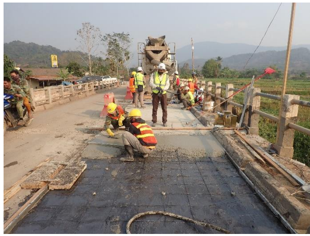
Compact Jet Concrete casting on Bridge Surface Span 2 R/S on 22 nd February 2023. (W= 2.70m, L= 19.3 m)
