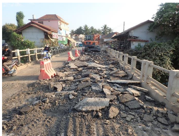
Removal of Existing pavement work on Bridge Surface Left side on 16 th February 2023
