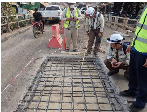
Install additional Reinforcing bar and Formwork on 18-19 th February 2023.
