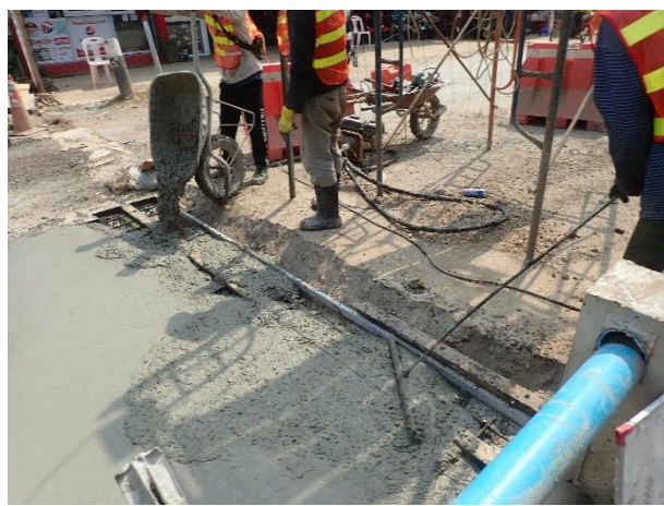
Compact Jet Concrete casting on Bridge Surface Span 1 L/S on 25 th February 2023. (SP 1 L/S: W= 3.25m, L= 11.95m)
