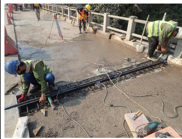
Installation of Expansion Joint at P1 L/S and A1 L/S on 24 th February 2023.
