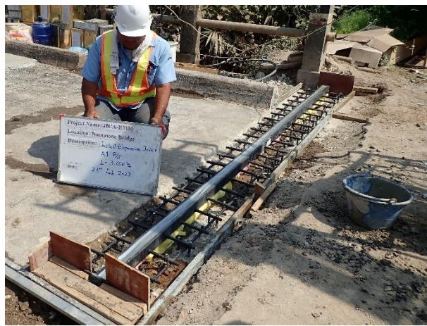
Installation of Expansion Joint (L= 3.65m) at A1 R/S on 23 rd February 2023.
