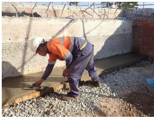
Leveling concrete under the Concrete Corbel on 23 rd December 2022.
