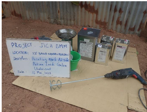
Under coat Patina Lock Galva PL-G on 16 th March 2023. Steel Girder web 3.00m, flange 7.00m, Steel Member, Handrail
