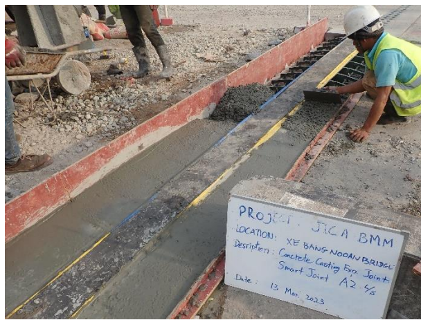
Casting Concrete of Expansion Joint at Abutment 2 Left side on 13 th March 2023
