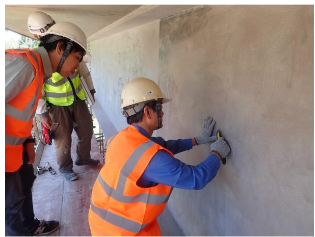
Preparation of the Steel Surface and Cleaning on 1-5 th March 2023. Steel Girder web 3.00m, flange 7.00m, Steel Member, Handrail
