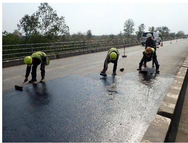
Apply Tack Coat (CRS-2) on Bridge Surface L/S on 1 st April 2023
