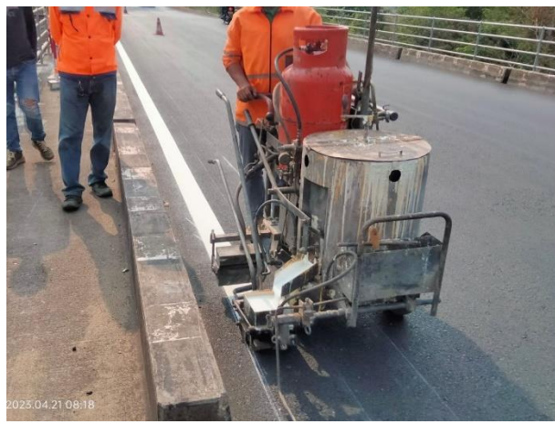
Edge line marking (Solid white line W=15cm) on Bridge Surface and Approach Road on 21 st April 2023
