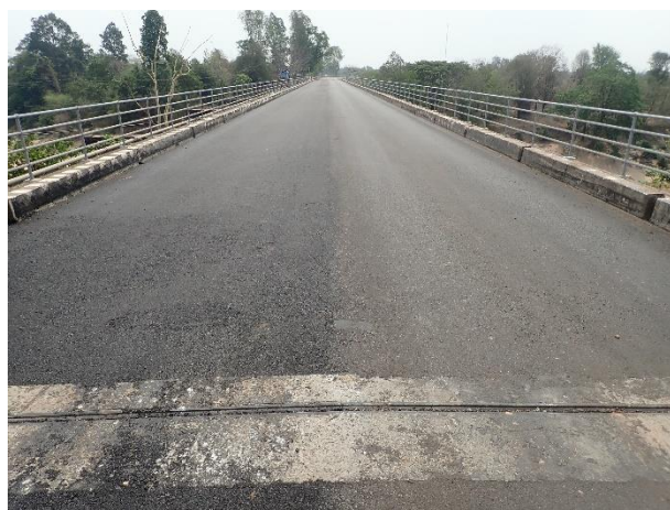
Completion of Asphalt pavement work on Bridge Surface 0 – 80 m from A1 side on 8 th April 2023
