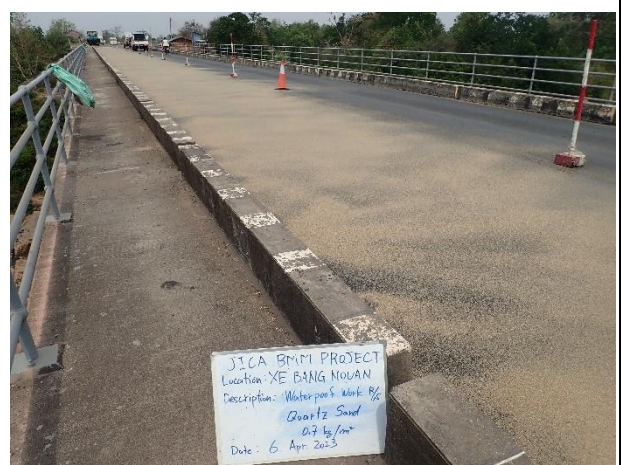
Sprinkle Quartz sand on Bridge Surface R/S on 6 th April 2023
