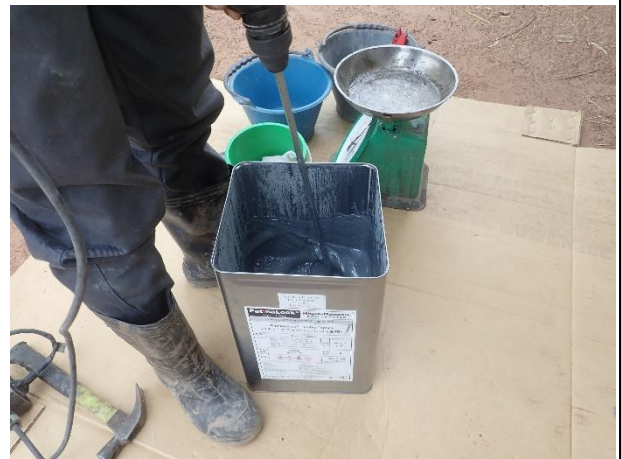
Under coat Patina Lock Galva PL-G on 16 th March 2023. Steel Girder web 3.00m, flange 7.00m, Steel Member, Handrail
