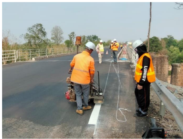
Edge line marking (Solid white line W=15cm) on Bridge Surface and Approach Road on 21 st April 2023
