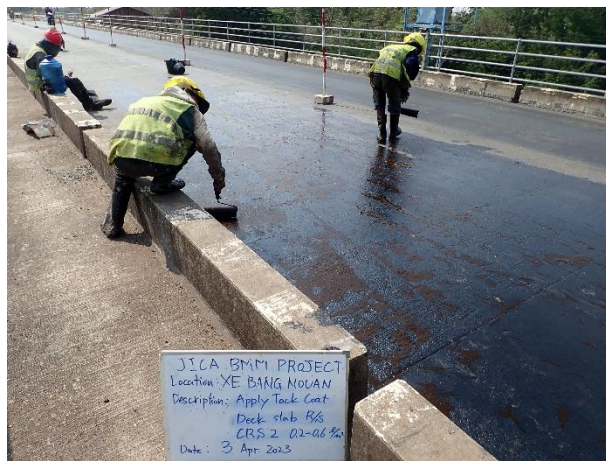
Apply Tack Coat (CRS-2) on Bridge Surface R/S on 3 rd April 2023
