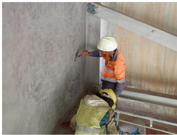
Under coat Patina Lock Galva PL-G on 16 th March 2023. Steel Girder web 3.00m, flange 7.00m, Steel Member, Handrail
