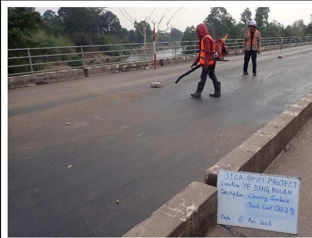
Cleaning Surface Tack coat (CRS-2) on Bridge Surface R/S on 6 th April 2023
