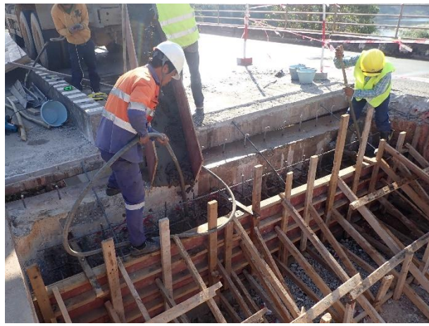
Concrete Casting for Concrete Corbel Abutment 1 Left side on 30 th December 2022.
