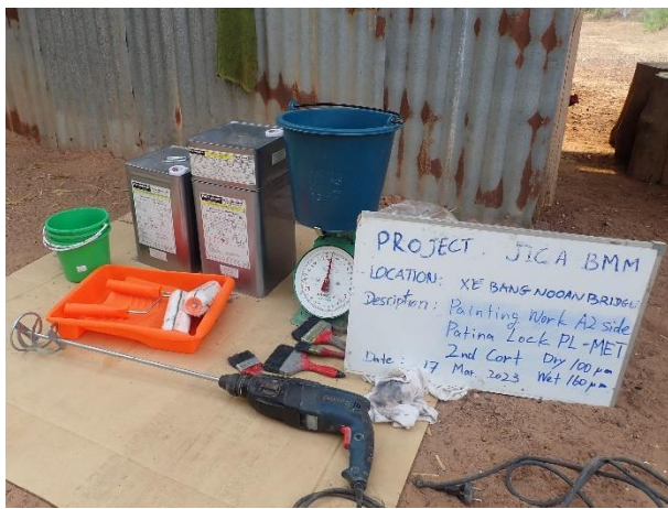
Second coat Patina Lock PL-MET on 17 th March 2023. Steel Girder web 3.00m, flange 7.00m, Steel Member, Handrail
