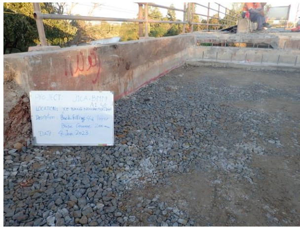
Backfilling by Crushed stone 4 th Layer on 4 th January 2023.
