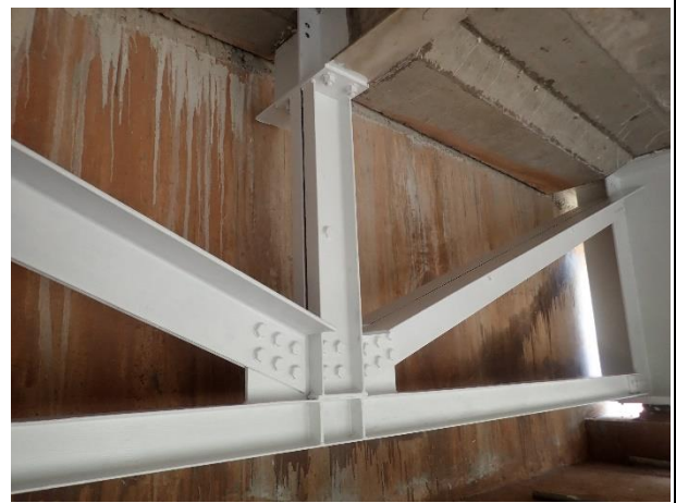
Second coat Patina Lock PL-MET on 17 th March 2023. Steel Girder web 3.00m, flange 7.00m, Steel Member, Handrail
