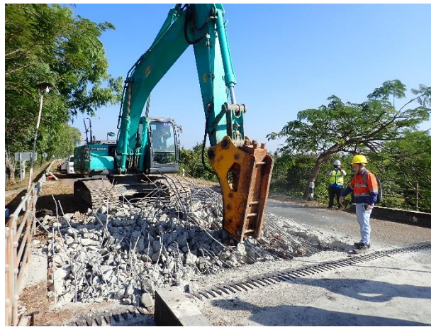
Removal of Existing pavement work on Approach Road Left side on 15-17 th December 2022
