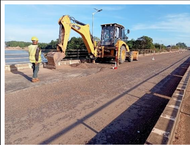
Removal of Existing pavement work on Bridge Surface on 25-30 th November 2022
