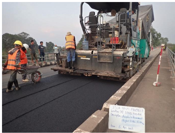
Asphalt pavement work on Bridge Surface R/S on 6 th April 2023
