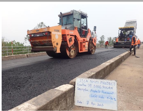
Asphalt pavement work on Bridge Surface L/S on 7 th April 2023
