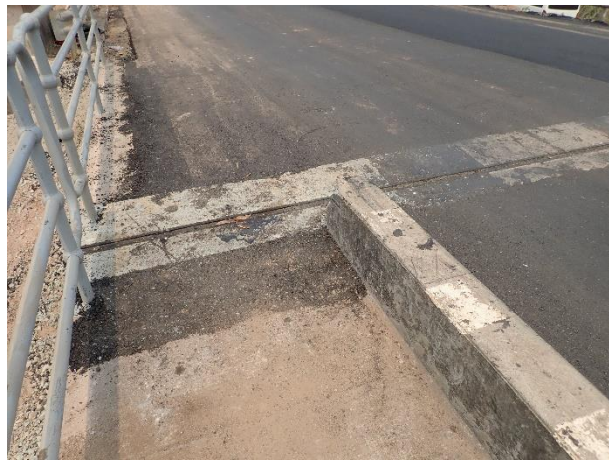
Completion of Asphalt pavement work at near the Expansion joint on 8 th April 2023
