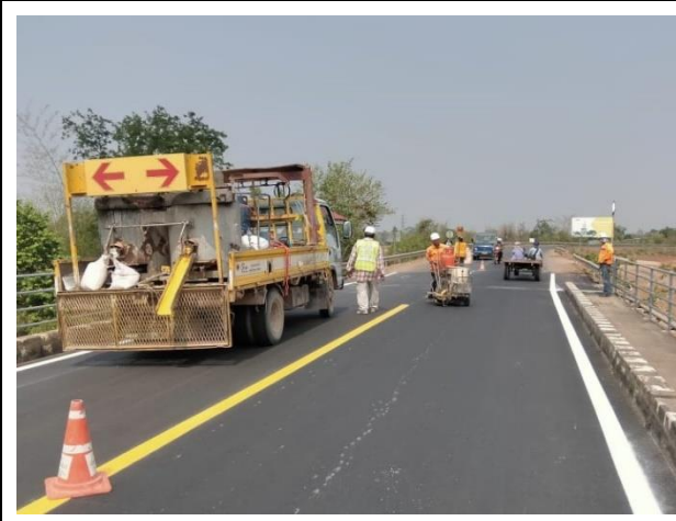
Center line marking (Solid yellow line W=15cm) on Bridge Surface and Approach Road on 21 st April 2023
