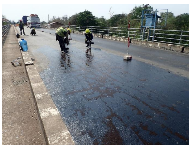
Apply Tack Coat (CRS-2) on Bridge Surface R/S on 3 rd April 2023
