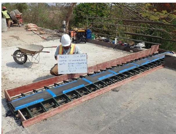
Installation of Expansion Joint at Abutment 2 Right side on 5 th March 2023
