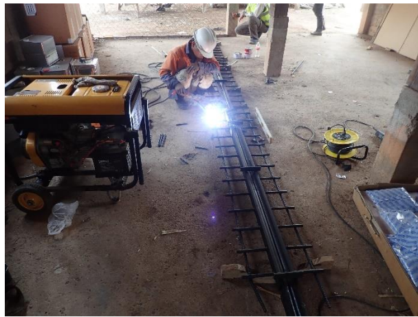
Assembly of Expansion Joint and cleaning work at Abutment 1 Left site on 8-9 th March 2023
