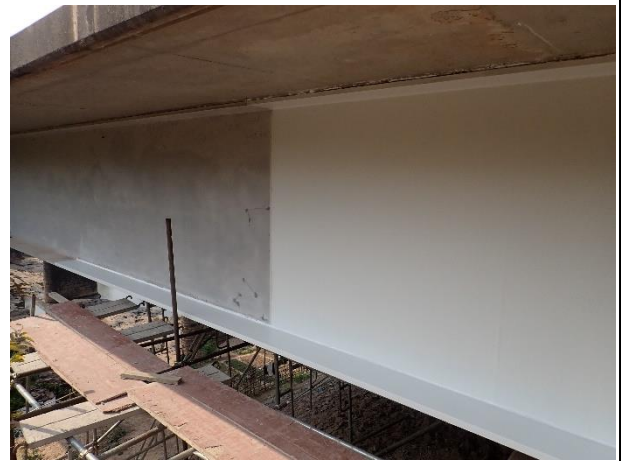
Second coat Patina Lock PL-MET on 17 th March 2023. Steel Girder web 3.00m, flange 7.00m, Steel Member, Handrail
