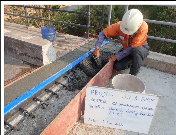
Casting Concrete of Expansion Joint at Abutment 1 Right side on 5 th March 2023
