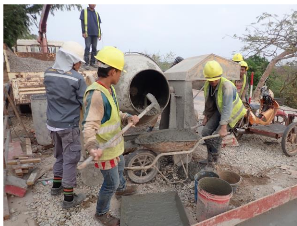
Concrete Mixing (Cement 25kg, Water 8.76kg, Fine Agg. 28.0kg, Course Agg. 51.66kg) with Admixture Sika plast-204L 0.24kg, Slump 18.5cm
