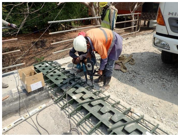
Installation of Expansion Joint at Abutment 2 Left side on 5 th March 2023
