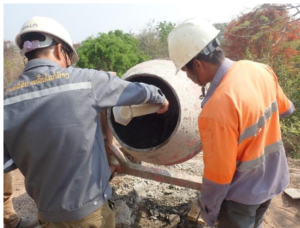
Concrete Mixing (Cement 50kg, Water 17.52kg, Fine Agg. 55.9kg, Course Agg. 103.33kg) with Admixture Sika plast-204L 0.48kg, Slump 13.0cm, Temperature 32°C
