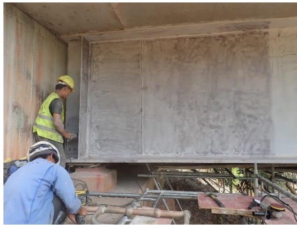
Preparation of the Steel Surface and Cleaning on 14 th March 2023. Steel Girder web 3.00m, flange 7.00m, Steel Member, Handrail
