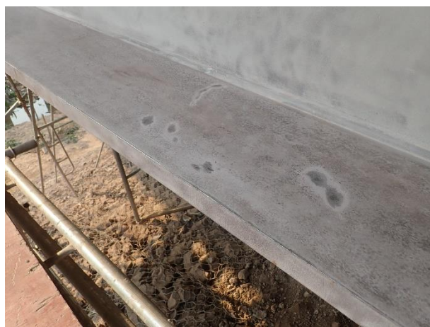
Preparation of the Steel Surface and Cleaning on 15 th March 2023. Steel Girder web 3.00m, flange 7.00m, Steel Member, Handrail
