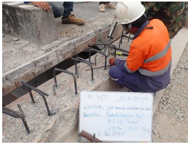
Install Anchor bar for Parapet work on 6 th January 2023.
