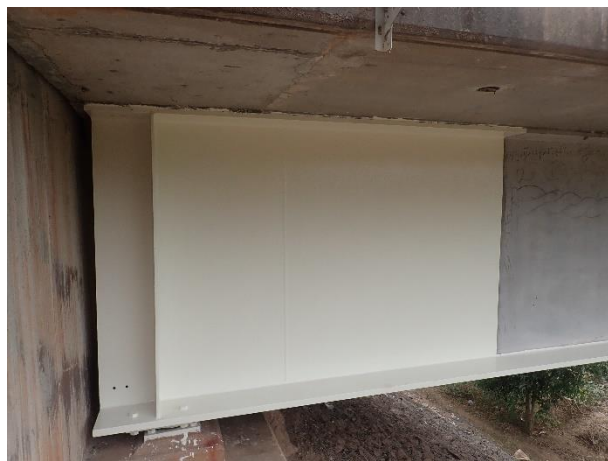
Completion of repainting work A2 side on 19 th March 2023.
