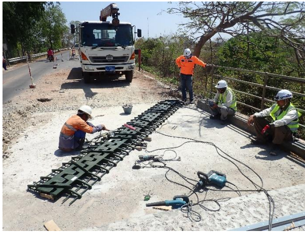
Assembly of Expansion Joint and setting at Abutment 2 Right side on 3-4 th March 2023
