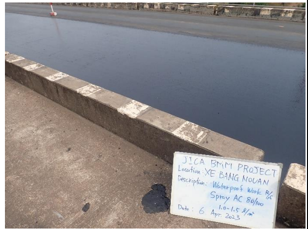
Splaying Bitumen AC 80/100 on Bridge Surface R/S on 6 th April 2023
