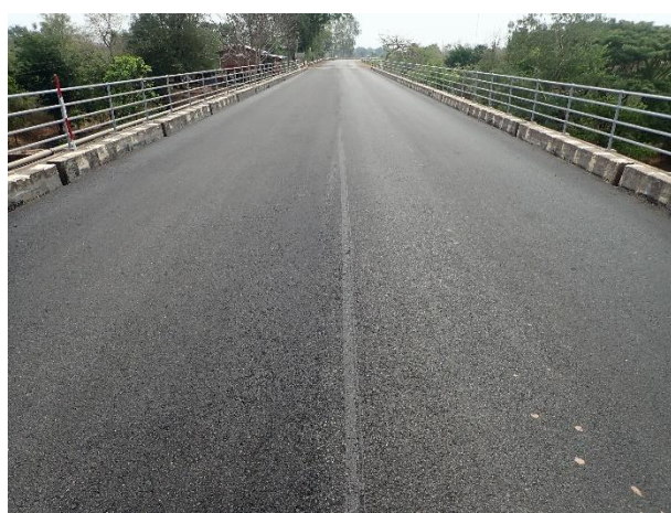
Completion of Asphalt pavement work on Bridge Surface 80 – 140 m from A1 side on 8 th April 2023
