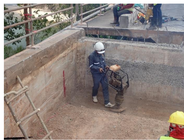
Foundation compaction work under the Concrete Corbel on 21 st December 2022.
