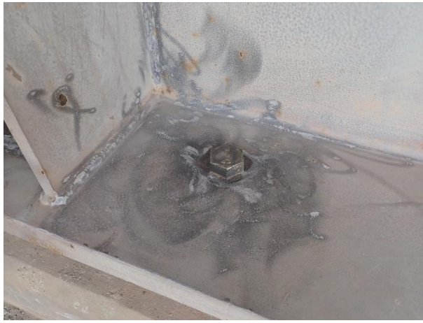
Preparation of the Steel Surface and Cleaning on 11 th March 2023.
