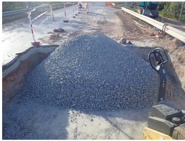
Backfilling by Crushed stone 4 th Layer on 4 th January 2023.
