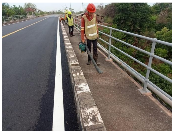
Cleaning and Apply EPS on Bridge Surface Footpath B/S on 24 th April 2023
