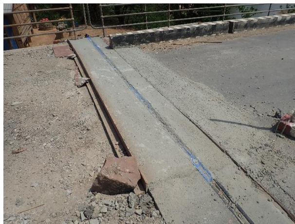
Completion Replacement of Expansion Joint at Abutment 1 site on 14 th March 2023
