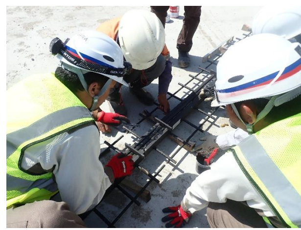
Assembly of Expansion Joint at Abutment 1 Right side on 2 nd March 2023
