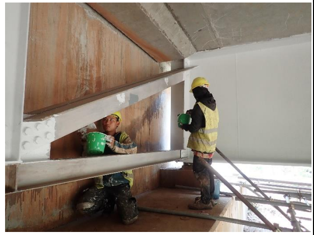
Second coat Patina Lock PL-MET on 17 th March 2023. Steel Girder web 3.00m, flange 7.00m, Steel Member, Handrail
