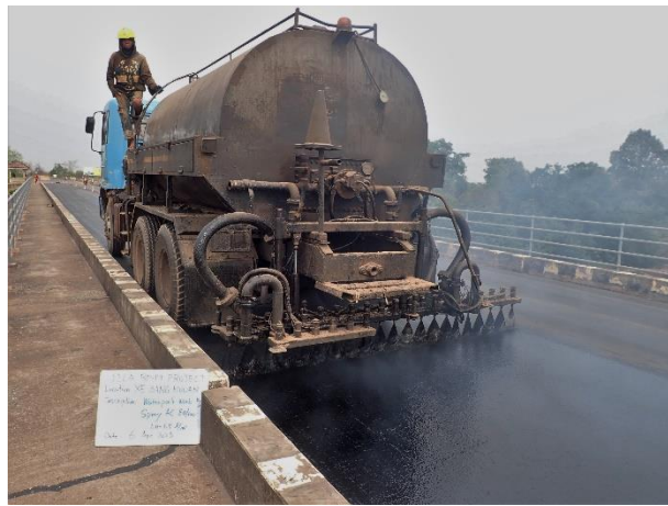
Splaying Bitumen AC 80/100 on Bridge Surface R/S on 6 th April 2023
