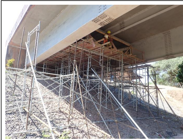
Scaffolding assembly and Cleaning work for the Steel Surface on 1-5 th March 2023. Steel Girder web 3.00m, flange 7.00m, Steel Member, Handrail
