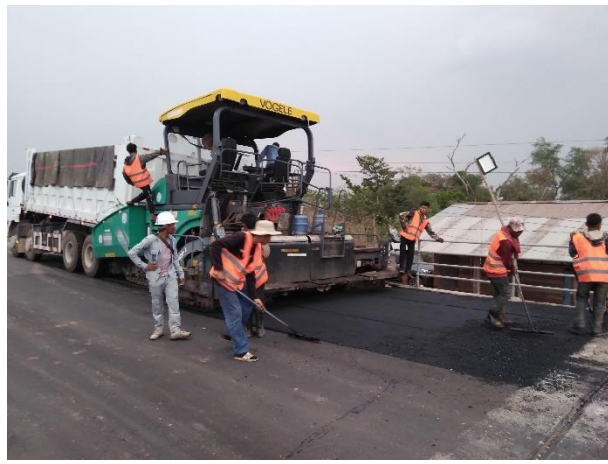
Asphalt pavement work on Approach road A1 L/S on 7 th April 2023
