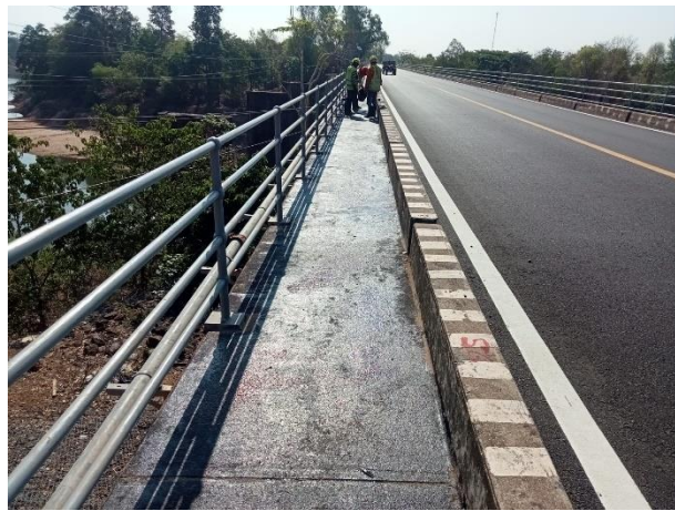
Apply Tack coat (CRS-2) and Sprinkle Quartz sand on Bridge Surface L/S on 25 th April 2023
