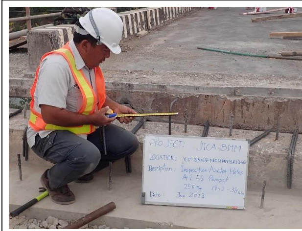
Inspection for Anchor holes for Parapet work on 6 th January 2023.
