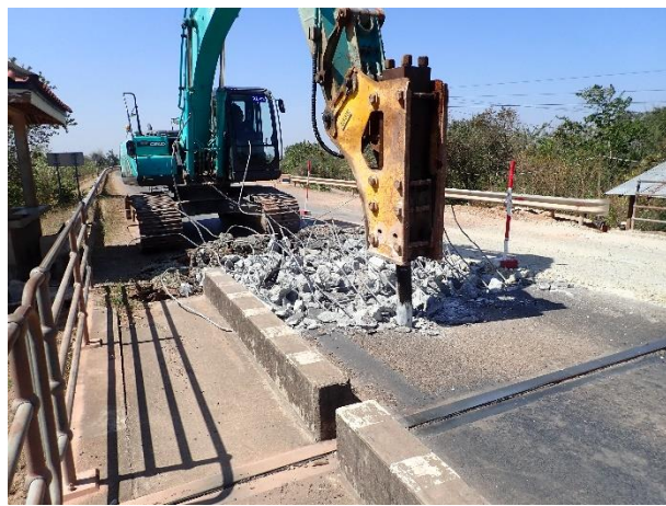
Removal of Existing pavement work on Approach Road Right side on 30 January -1 st February 2023
