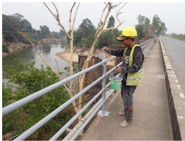
Painting work with TERMARUST on 19-20 th March 2023. Handrail 145m, Both side
