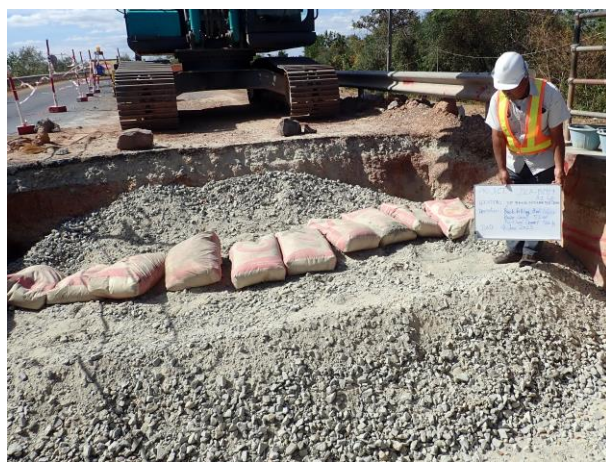
Backfilling by Soil cement 3 rd Layer on 4 th January 2023.
