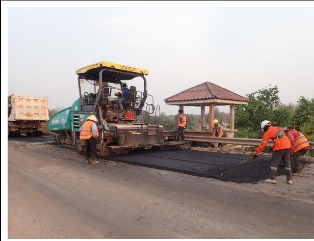
Asphalt pavement work on Approach road A1 R/S on 6 th April 2023
