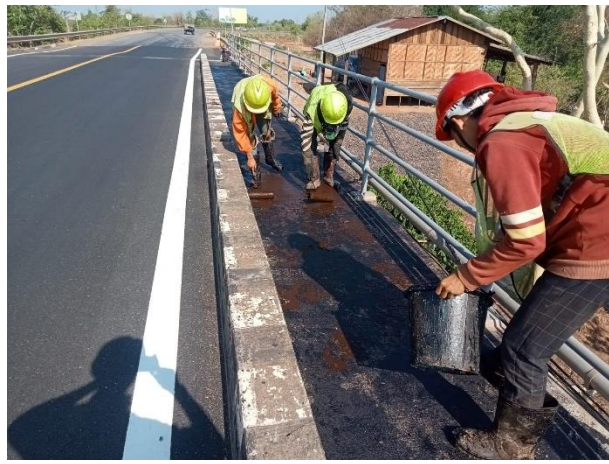
Apply Tack coat (CRS-2) on Bridge Surface Footpath B/S on 25 th April 2023
