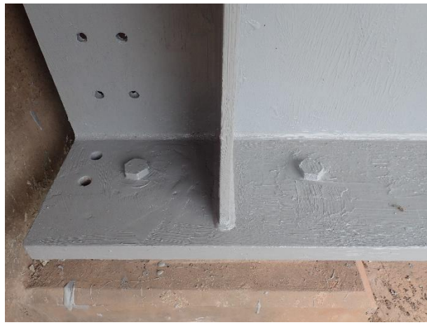
Painting work with TERMARUST on 11-12 th March 2023. Steel Girder web 3.00m, flange 7.00m, Steel Member
