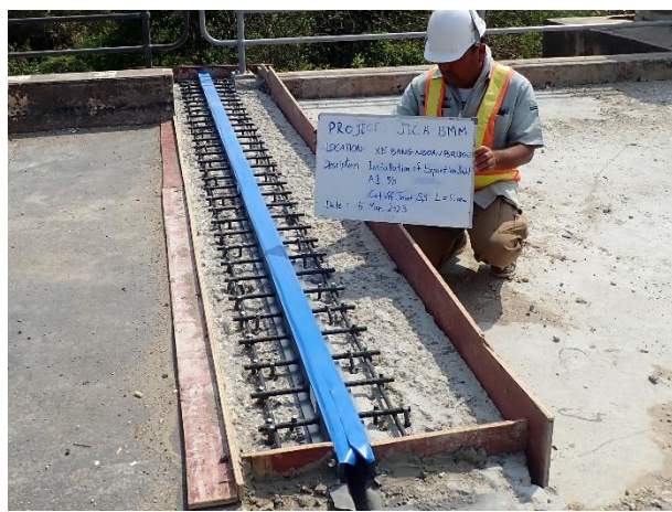
Installation of Expansion Joint at Abutment 1 Right side on 5 th March 2023
