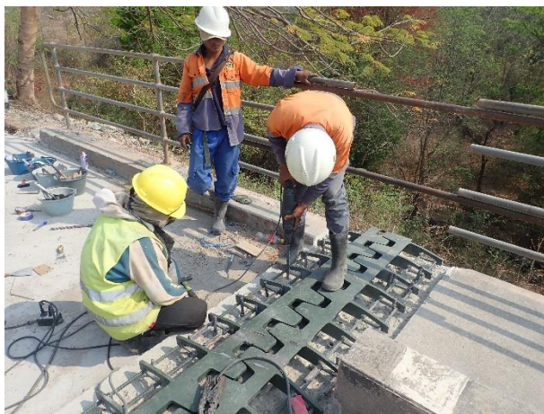
Installation of Expansion Joint at Abutment 2 Right side on 4 th March 2023
