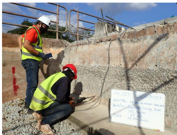
Concrete Drilling work for anchor holes on 24-28 th December 2022.
