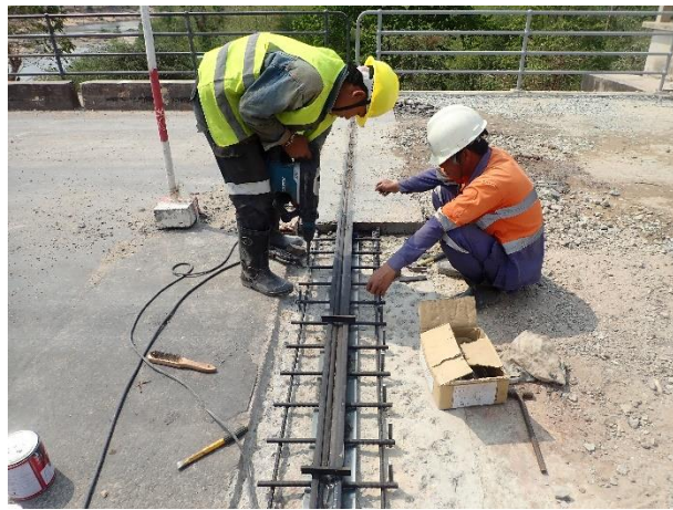
Installation of Expansion Joint at Abutment 1 Left site on 9 th March 2023
