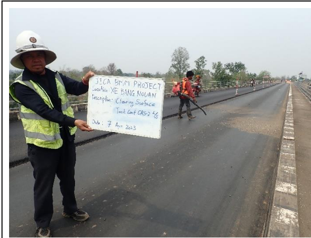
Cleaning Surface Tack coat (CRS-2) on Bridge Surface L/S on 7 th April 2023
