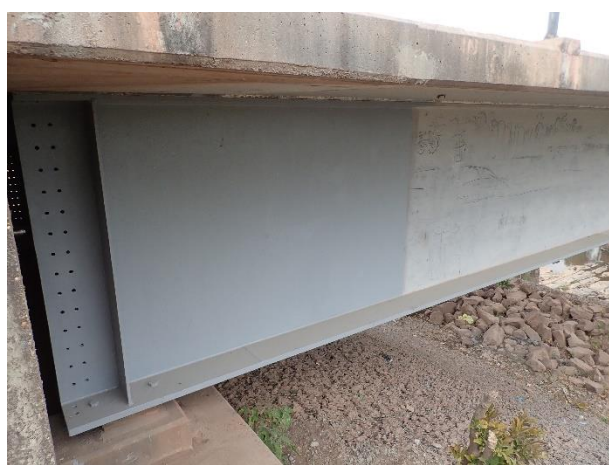
Completion of repainting work A1 side on 19 th March 2023. Steel Girder web 3.00m, flange 7.00m, Steel Member
