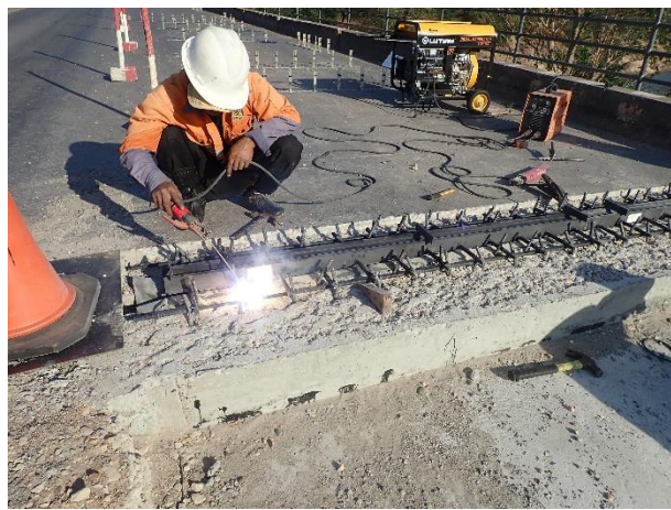
Installation of Expansion Joint at Abutment 1 Right side on 3 rd March 2023
