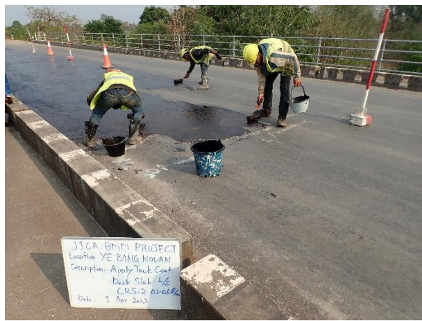
Apply Tack Coat (CRS-2) on Bridge Surface L/S on 1 st April 2023
