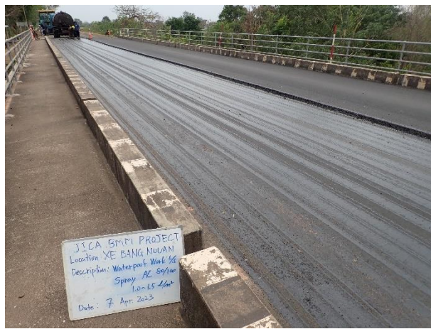
Splaying Bitumen AC 80/100 on Bridge Surface L/S on 7 th April 2023
