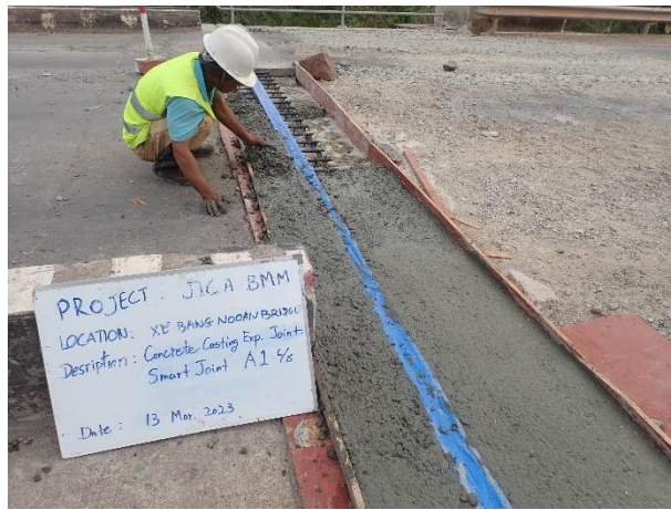
Casting Concrete of Expansion Joint at Abutment 1 Left site on 13 th March 2023
