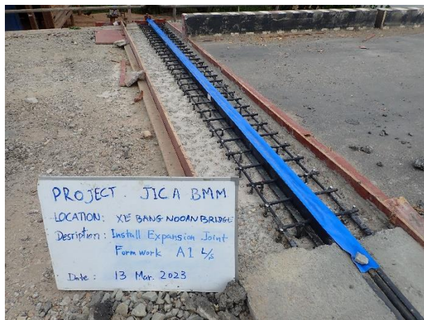
Installation of Expansion Joint and Formwork at Abutment 1 Left site on 13 th March 2023
