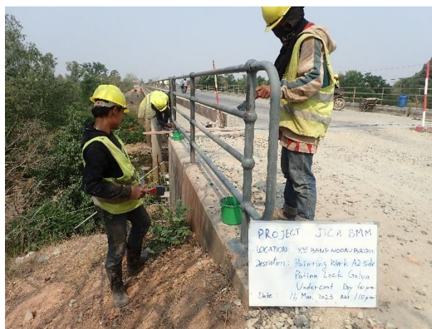
Under coat Patina Lock Galva PL-G on 16 th March 2023. Steel Girder web 3.00m, flange 7.00m, Steel Member, Handrail
