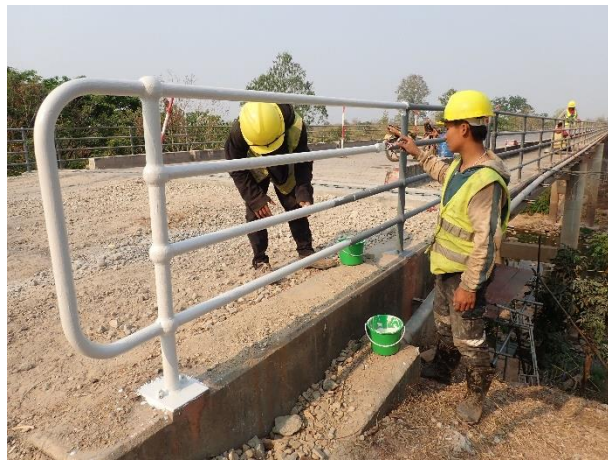
Second coat Patina Lock PL-MET on 17 th March 2023. Steel Girder web 3.00m, flange 7.00m, Steel Member, Handrail
