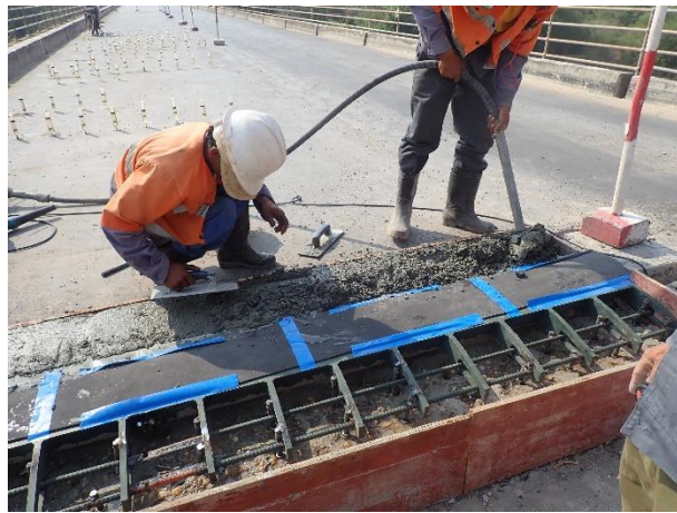
Casting Concrete of Expansion Joint at Abutment 2 Right side on 5 th March 2023
