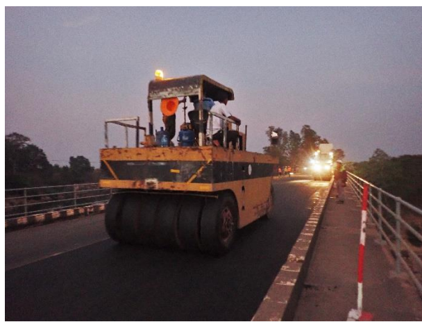
Asphalt pavement work on Bridge Surface R/S on 6 th April 2023
