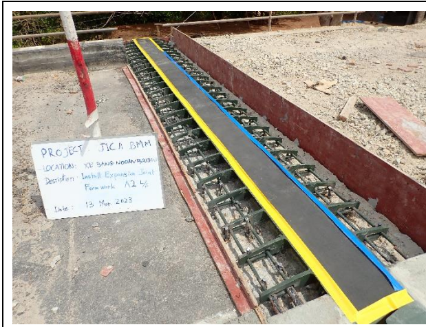
Installation of Expansion Joint and Formwork at Abutment 2 Left side on 13 th March 2023
