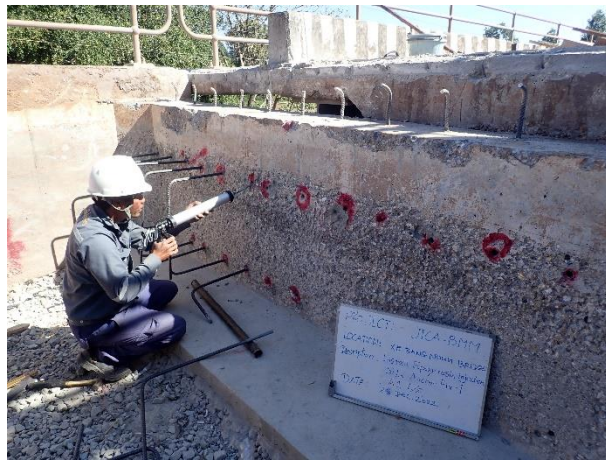
Anchor rebar insert to Existing concrete wall on 28 th December 2022.
