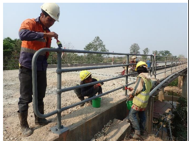
Under coat Patina Lock Galva PL-G on 16 th March 2023. Steel Girder web 3.00m, flange 7.00m, Steel Member, Handrail
