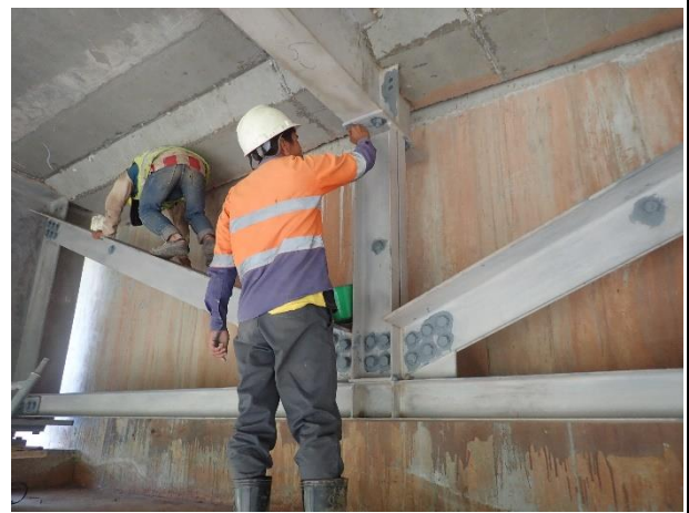
Under coat Patina Lock Galva PL-G on 16 th March 2023. Steel Girder web 3.00m, flange 7.00m, Steel Member, Handrail
