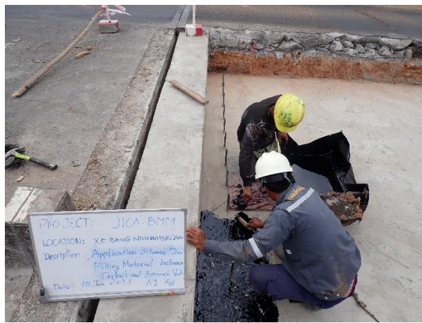
Application Bitumen 80/100 as filling material between Corbel and Approach slab on 10 th January 2023.
