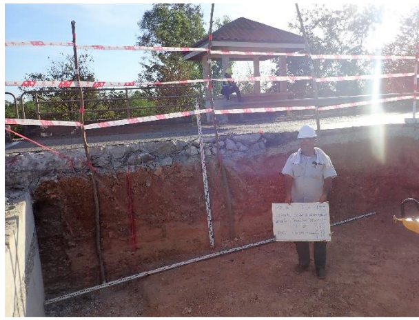
Completion of Excavation work under the Approach slab on 20 th December 2022. Upper: L=6.00m, W=4.80m, Lower: L=5.50m W=4.65m, H 1 =1.75m, H 2 =1.55m
