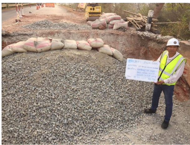
Backfilling by Soil cement 1 st Layer on 14 th February 2023.
