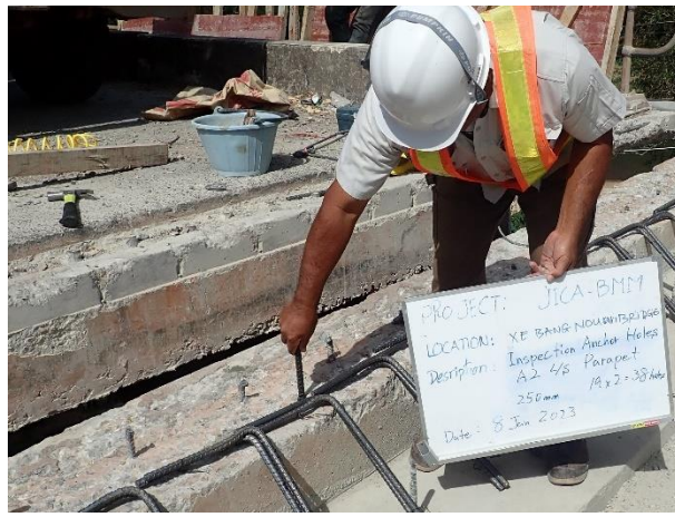
Inspection for Anchor holes for Parapet work on 8 th January 2023.
