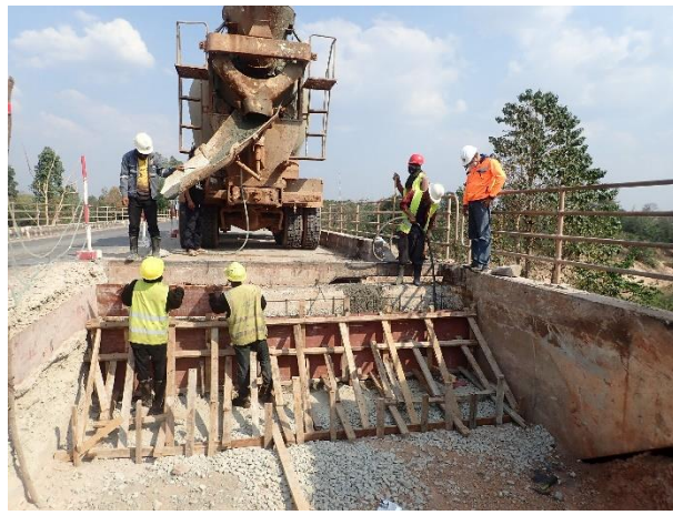
Concrete Casting for Concrete Corbel Abutment 1 Right side on 10 th February 2023.
