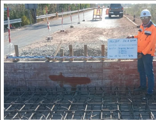
Inspection for Form work and Anchor cap setting on 24 th February 2023.
