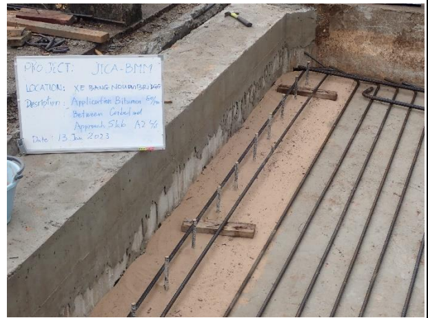
Application Bitumen 80/100 as filling material between Corbel and Approach slab on 13 th January 2023.
