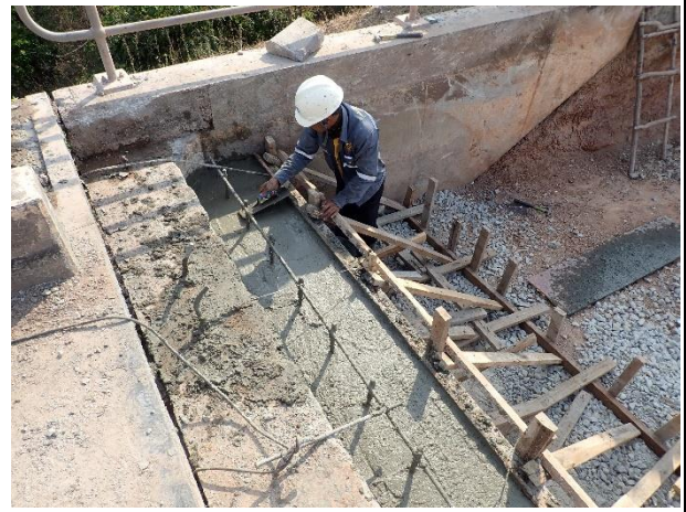
Concrete Casting for Concrete Corbel Abutment 1 Right side on 10 th February 2023.
