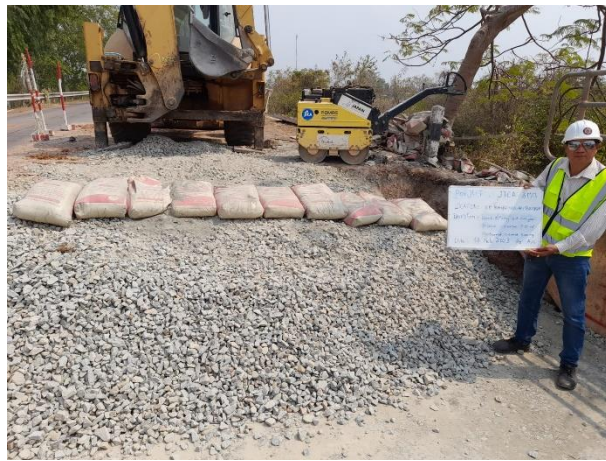
Backfilling by Soil cement 3 rd Layer and Crushed stone 4 th Layer on 14 th February 2023. Base course 5.0 m 3 + Portland Cement 500kg, Base course 5.5 m 3
