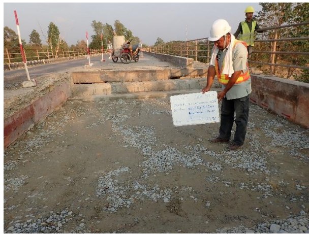
Backfilling by Crushed stone 4 th Layer on 12 th February 2023.
