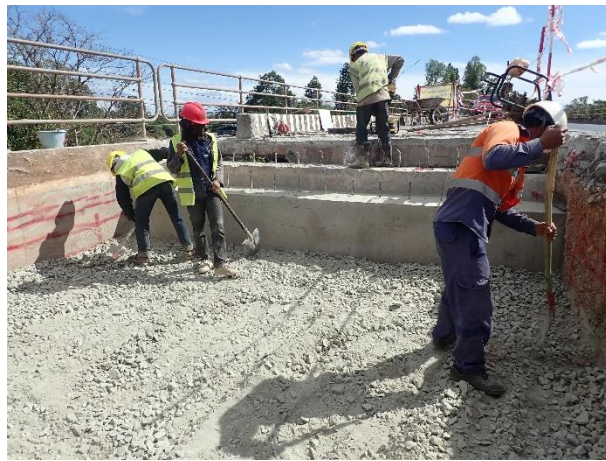
Backfilling by Soil cement 2 nd Layer on 4 th January 2023.
