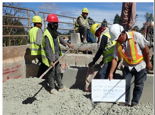
Backfilling by Soil cement 3 rd Layer on 4 th January 2023.
