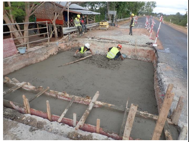
Leveling concrete under the Approach slab on 9 th January 2023.
