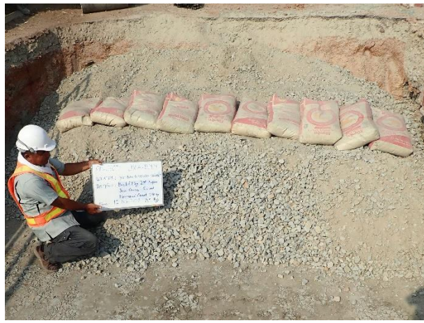
Backfilling by Soil cement 2 nd Layer on 12 th February 2023.
