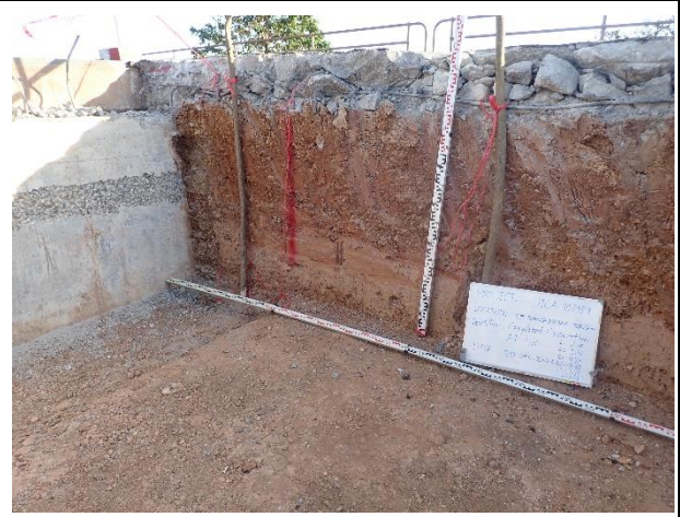
Completion of Excavation work under the Approach slab on 20 th December 2022. Upper: L=6.00m, W=4.80m, Lower: L=5.50m W=4.65m, H 1 =1.75m, H 2 =1.55m
