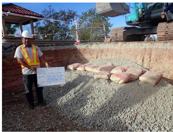
Backfilling by Soil cement 1 st Layer on 4 th January 2023. Base course 5.0 m 3 + Portland Cement 500kg
