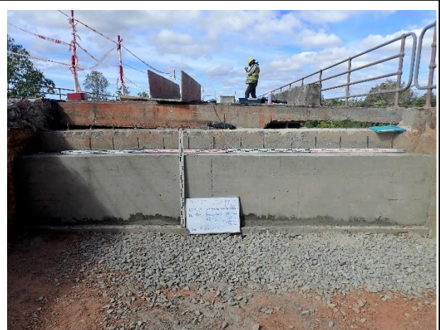
Inspection for Concrete Corbel Abutment 2 Left side on 5 th January 2023. L=505mm, W=4650mm, H=800mm
