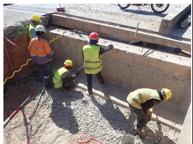
Concrete Drilling work for anchor holes on 23-29 th December 2022.
