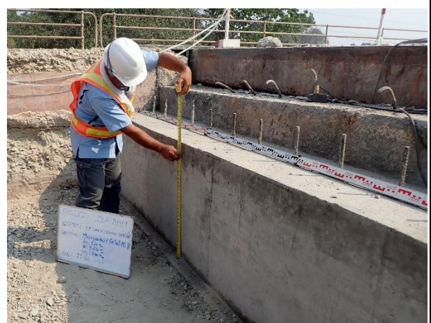
Inspection for Concrete Corbel Abutment 1 Right side on 11 th February 2023. L=520mm, W=4650mm, H=800mm
