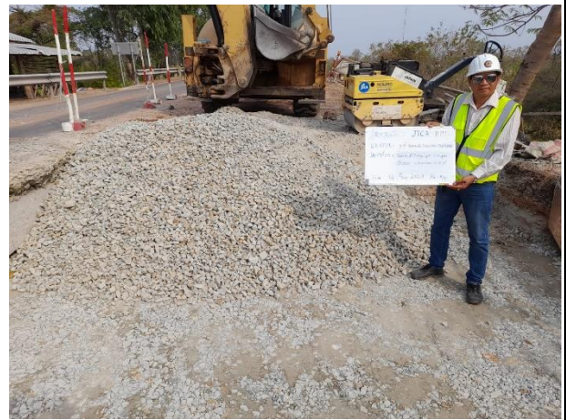
Backfilling by Soil cement 3 rd Layer and Crushed stone 4 th Layer on 14 th February 2023. Base course 5.0 m 3 + Portland Cement 500kg, Base course 5.5 m 3
