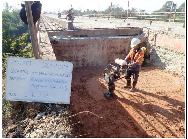
Excavation and Compaction work under the Approach slab on 1 st February 2023.
