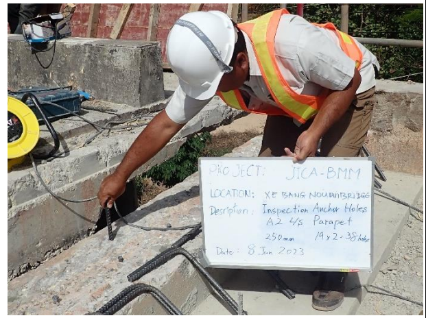
Inspection for Anchor holes for Parapet work on 8 th January 2023.
