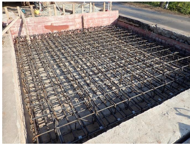
Inspection for Re-bar work on 14 th January 2023.
