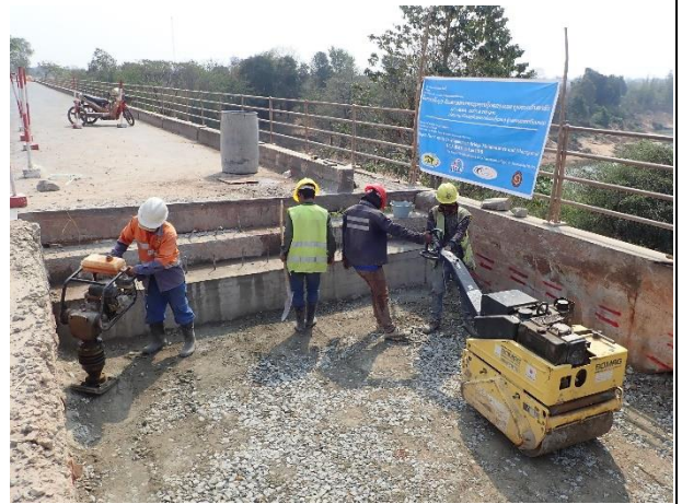
Backfilling by Soil cement 2 nd Layer on 12 th February 2023.
