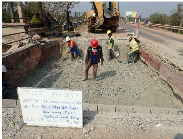
Backfilling by Soil cement 2 nd Layer on 12 th February 2023.
