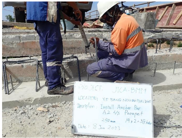
Install Anchor bar for Parapet work on 8 th January 2023.
