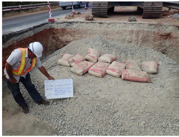
Backfilling by Soil cement 2 nd Layer on 4 th January 2023.
