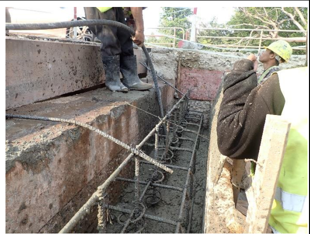
Concrete Casting for Concrete Corbel Abutment 2 Right side on 10 th February 2023.
