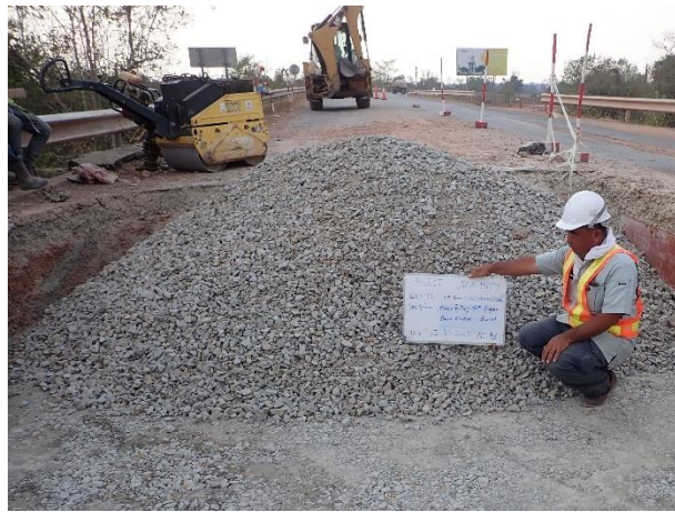
Backfilling by Crushed stone 4 th Layer on 12 th February 2023.
