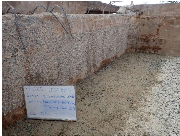
Foundation compaction work under the Concrete Corbel and Formwork on 3 rd February 2023.
