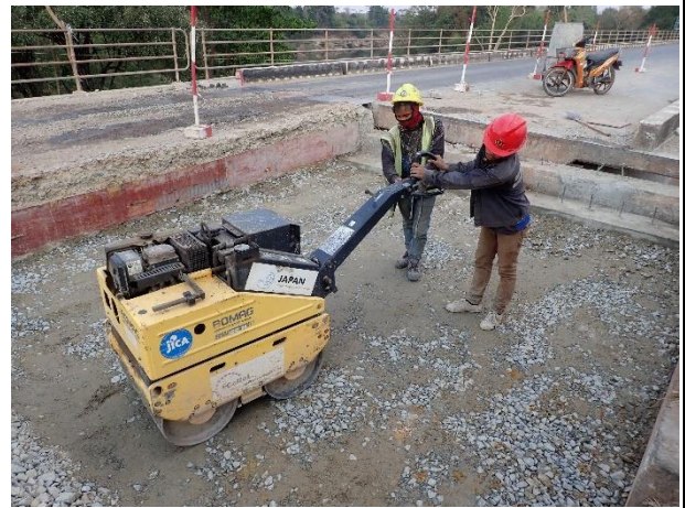
Backfilling by Crushed stone 4 th Layer on 12 th February 2023.
