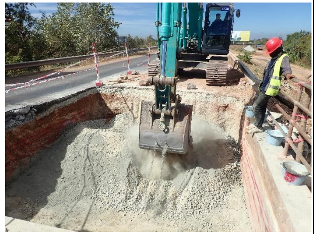
Backfilling by Soil cement 2 nd Layer on 4 th January 2023.
