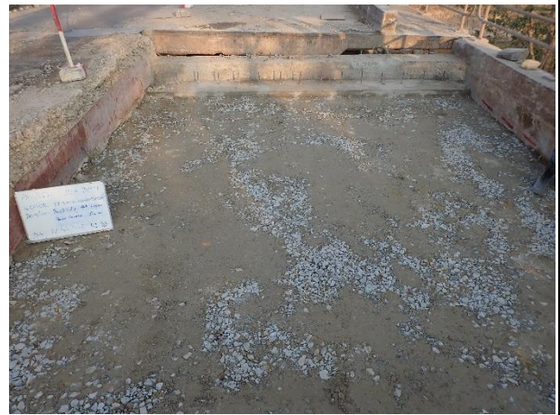
Backfilling by Crushed stone 4 th Layer on 12 th February 2023.
