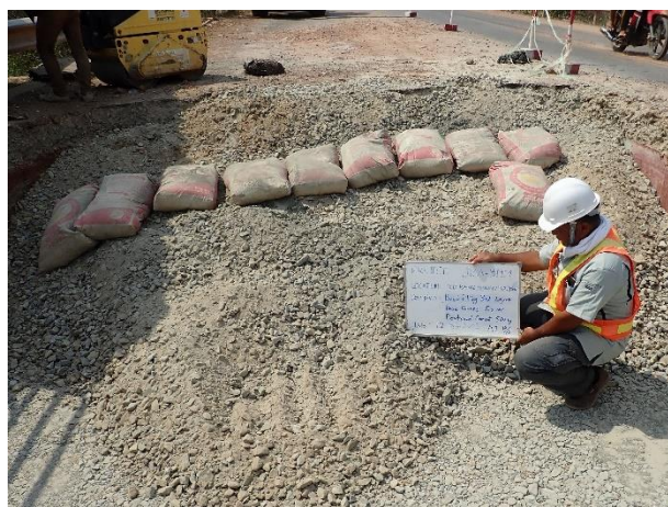
Backfilling by Soil cement 3 rd Layer on 12 th February 2023.
