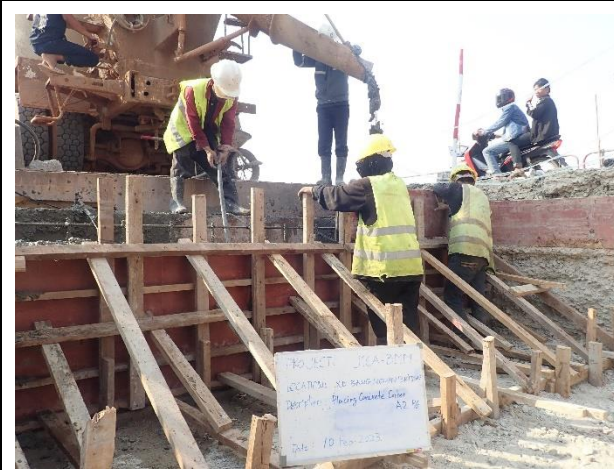
Concrete Casting for Concrete Corbel Abutment 2 Right side on 10 th February 2023.
