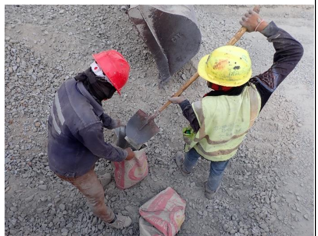
Backfilling by Soil cement 3 rd Layer on 12 th February 2023.
