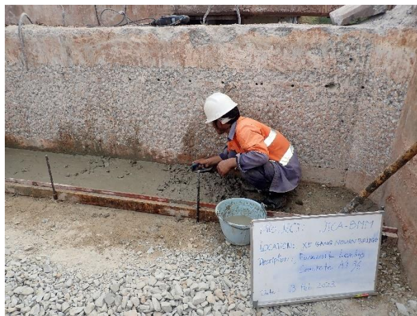
Leveling concrete under the Concrete Corbel on 3 rd February 2023.
