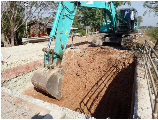
Excavation and Compaction work under the Approach slab on 1 st February 2023.
