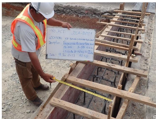
Inspection for Re-bar and Form work on 9 th January 2023.
