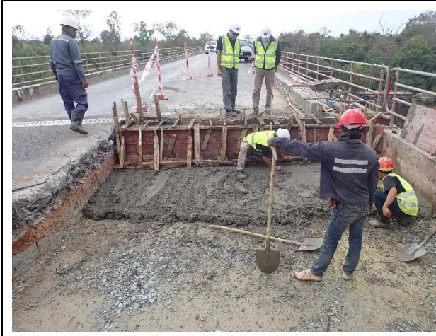
Leveling concrete under the Approach slab on 9 th January 2023.
