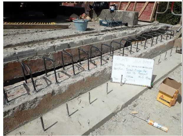
Install Anchor bar for Parapet work on 8 th January 2023.
