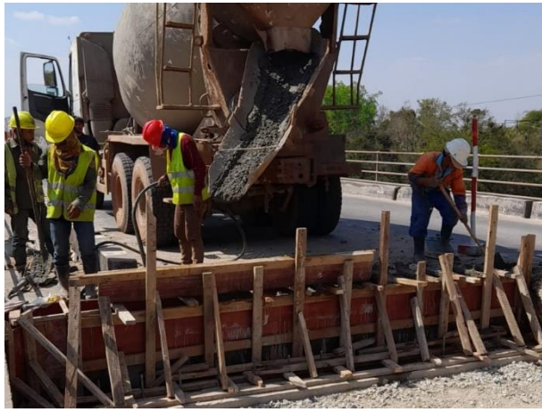
Concrete casting work on 17 th February 2023.
