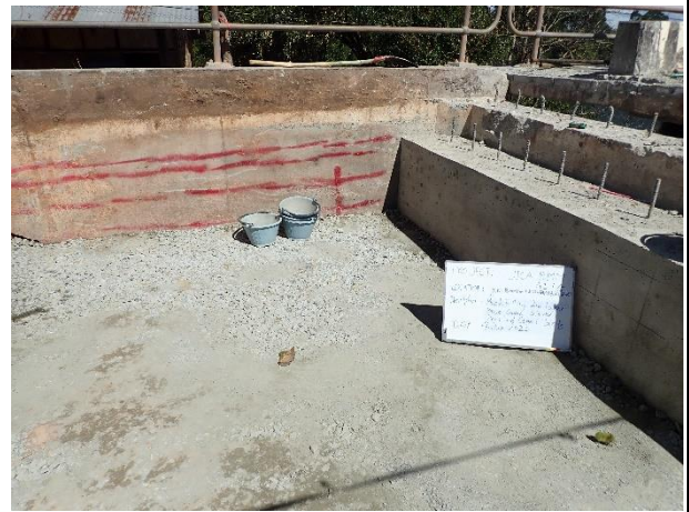
Backfilling by Soil cement 2 nd Layer on 4 th January 2023.
