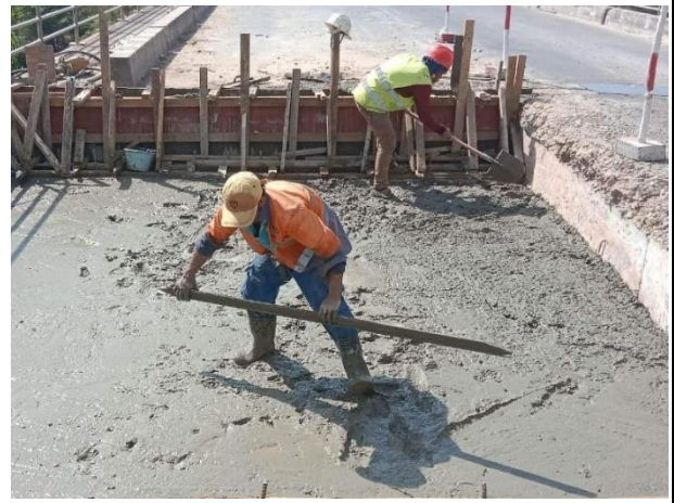
Leveling concrete under the Approach slab on 17 th February 2023.
