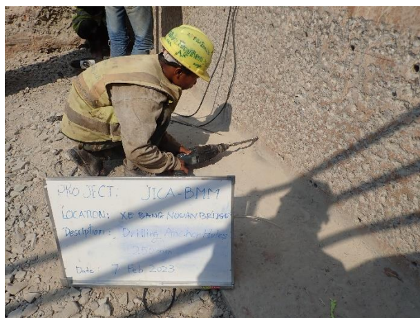
Concrete Drilling work for anchor holes on 7-8 th February 2023.
