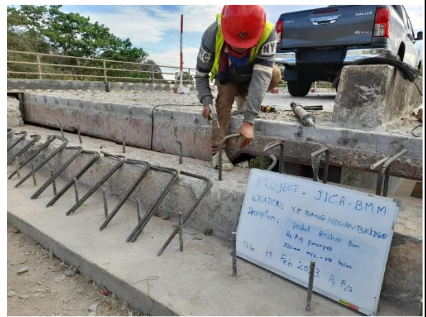
Install Anchor bar for Parapet work on 15 th February 2023.
