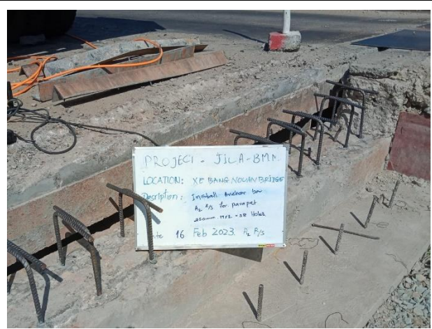
Inspection for Anchor holes for Parapet work on 16 th February 2023.
