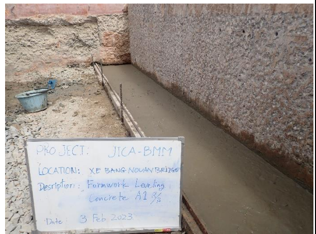
Leveling concrete under the Concrete Corbel on 3 rd February 2023.
