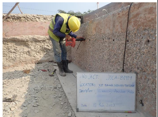
Concrete Drilling work for anchor holes on 7-8 th February 2023.
