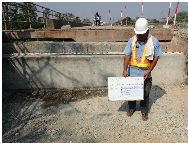
Inspection for Concrete Corbel Abutment 2 Right side on 11 th February 2023. L=500mm, W=4650mm, H=805mm
