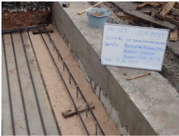
Application Bitumen 80/100 as filling material between Corbel and Approach slab on 13 th January 2023.
