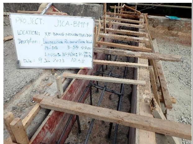
Inspection for Re-bar and Form work on 9 th January 2023.
