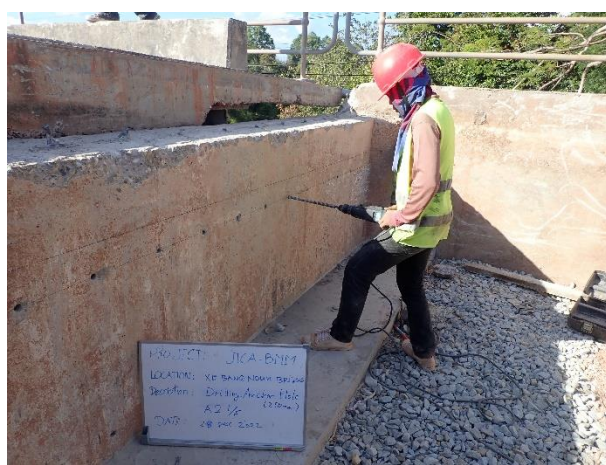
Concrete Drilling work for anchor holes on 23-29 th December 2022.
