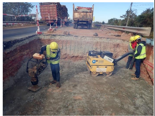
Backfilling by Soil cement 1 st Layer on 4 th January 2023. Base course 5.0 m 3 + Portland Cement 500kg
