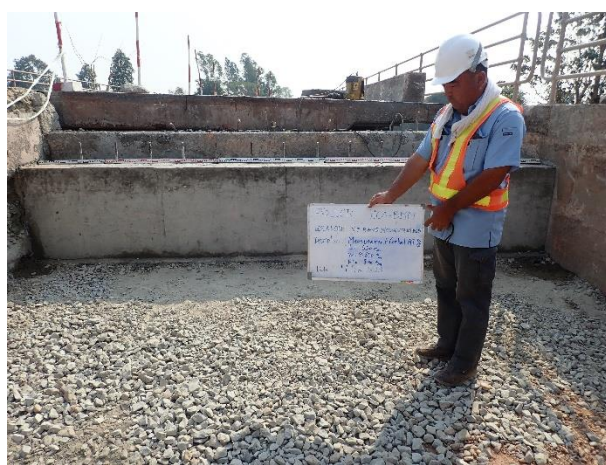
Inspection for Concrete Corbel Abutment 1 Right side on 11 th February 2023. L=520mm, W=4650mm, H=800mm
