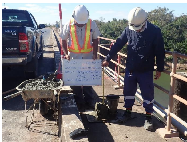
Concrete Casting for Concrete Corbel Abutment 2 Left side on 3 rd January 2023. Slump test 11.5 cm, Concrete Temperature 30 °C
