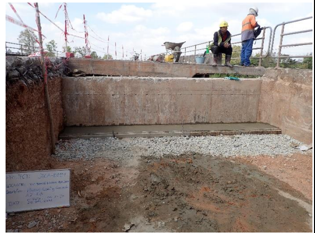
Leveling concrete under the Concrete Corbel on 24 th December 2022.
