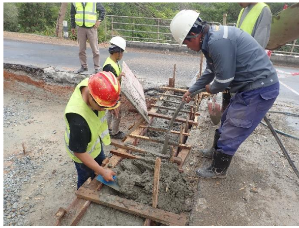
Concrete casting work on 9 th January 2023. Slump test 9.0 cm, Concrete Temperature 34.0 °C
