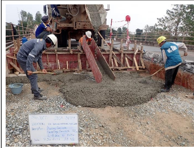
Leveling concrete under the Approach slab on 4 th January 2023.
