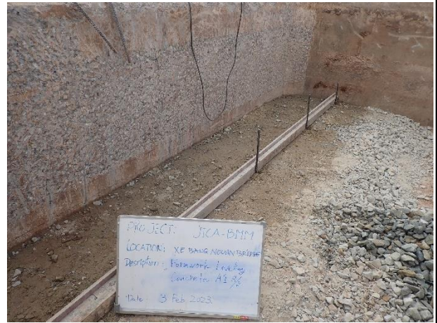
Foundation compaction work under the Concrete Corbel and Formwork on 3 rd February 2023.
