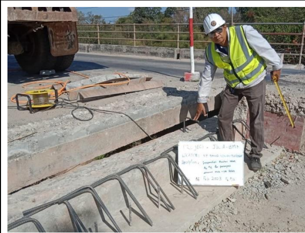
Inspection for Anchor holes for Parapet work on 16 th February 2023.
