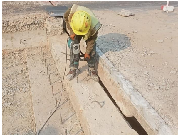
Inspection for Anchor holes for Parapet work on 15 th February 2023.
