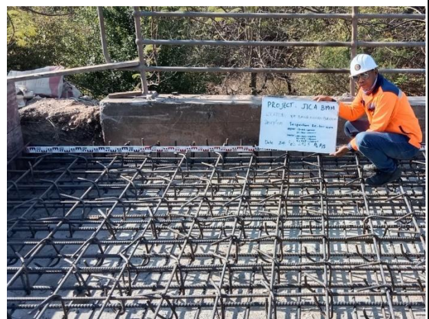
Inspection for Re-bar work on 24 th February 2023.
