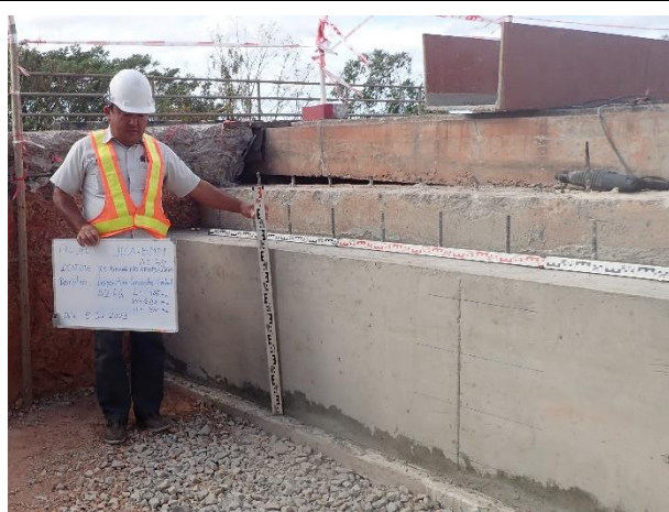
Inspection for Concrete Corbel Abutment 2 Left side on 5 th January 2023. L=505mm, W=4650mm, H=800mm
