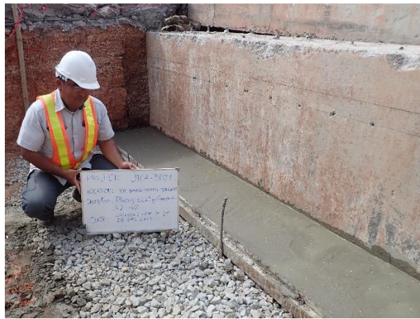
Leveling concrete under the Concrete Corbel on 24 th December 2022.
