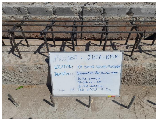
Inspection for Re-bar work on 15 th February 2023.
