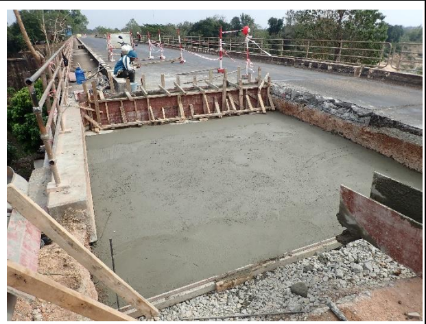
Leveling concrete under the Approach slab on 4 th January 2023.
