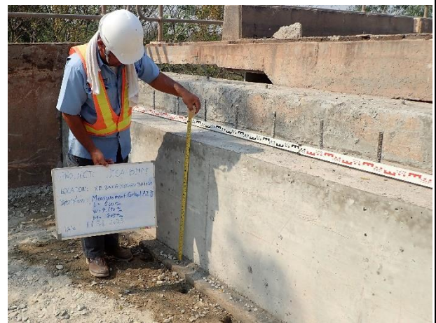
Inspection for Concrete Corbel Abutment 2 Right side on 11 th February 2023. L=500mm, W=4650mm, H=805mm
