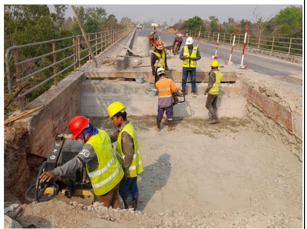
Backfilling by Soil cement 1 st Layer on 14 th February 2023.
