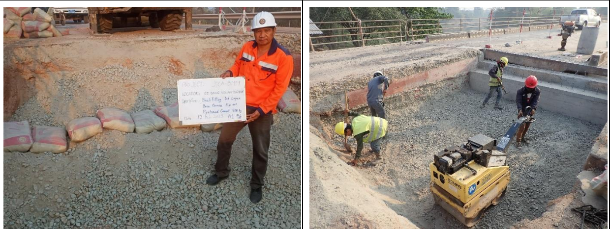
Backfilling by Soil cement 1 st Layer on 12 th February 2023.
