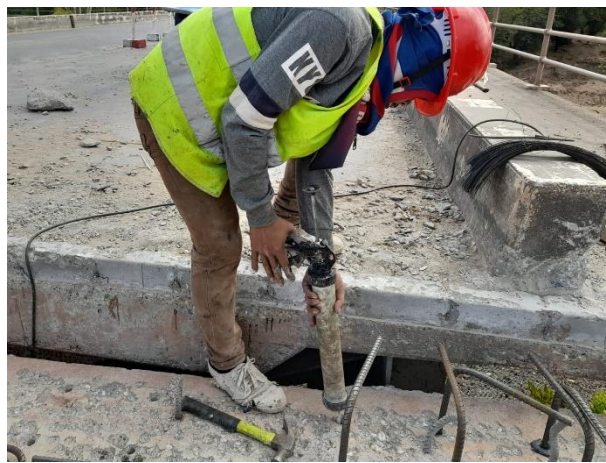
Install Anchor bar for Parapet work on 15 th February 2023.
