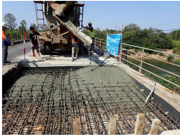
Concrete casting on 16 th January 2023.
