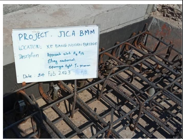
Inspection for Form work and Anchor cap setting on 24 th February 2023.
