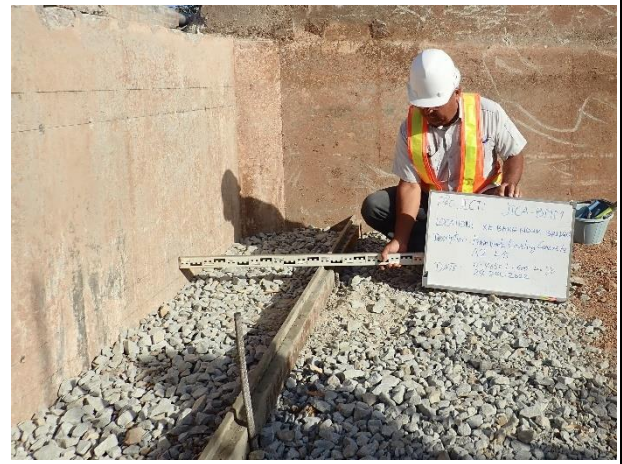
Leveling concrete under the Concrete Corbel on 24 th December 2022.
