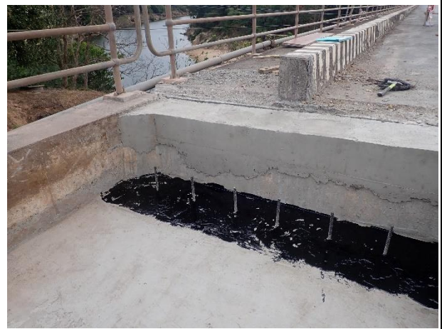
Application Bitumen 80/100 as filling material between Corbel and Approach slab on 10 th January 2023.
