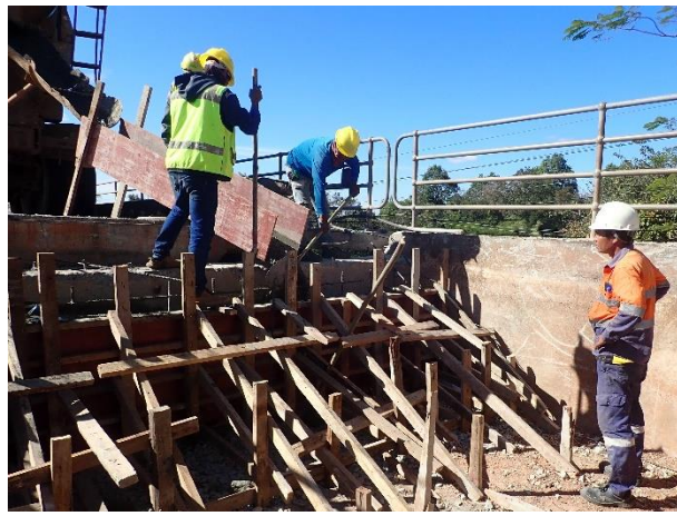
Concrete Casting for Concrete Corbel Abutment 2 Left side on 3 rd January 2023.
