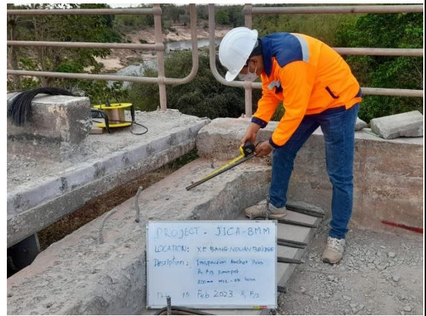
Inspection for Anchor holes for Parapet work on 15 th February 2023.
