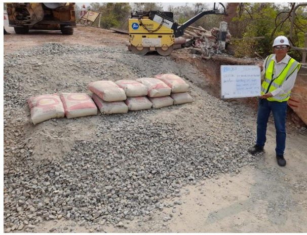
Backfilling by Soil cement 2 nd Layer on 14 th February 2023. Base course 5.0 m 3 + Portland Cement 500kg(Take a Test Sample)
