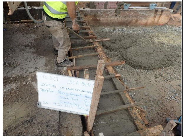
Concrete casting work on 9 th January 2023. Slump test 9.0 cm, Concrete Temperature 34.0 °C
