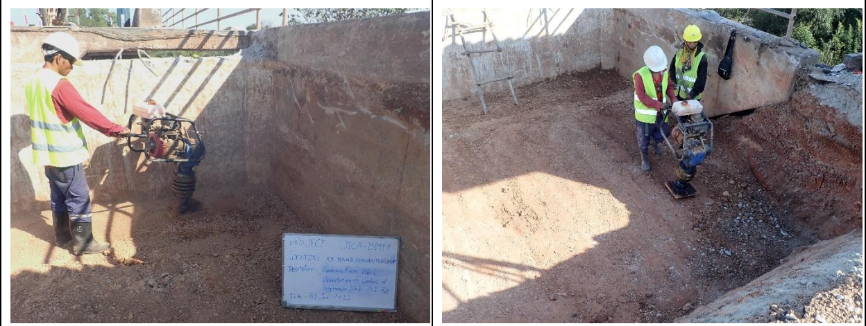
Compaction work under the Approach slab on 31 st January 2023.
