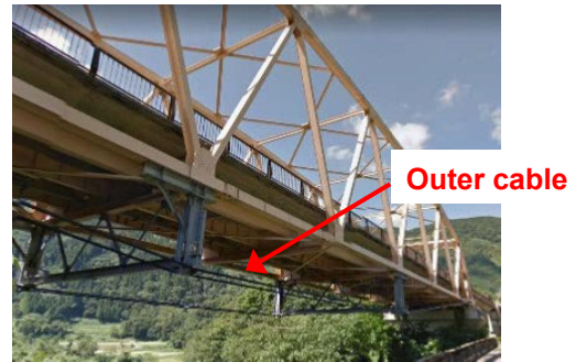
Example of a steel bridge reinforced with outer cables
