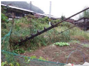
Anchoring with wire clip
