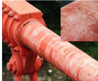
Galvanizing + Wrapping wire + Painting
