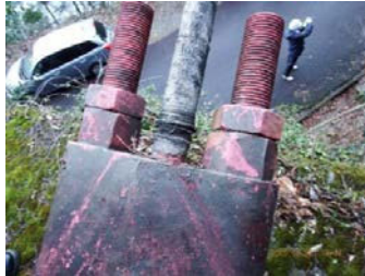
Anchoring to the anchor frame
