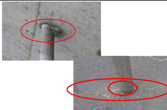
Deformation that suggests internal corrosion
