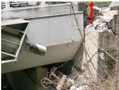
Lifting out of the girder
