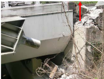
Lifting out of the girder
