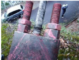
Anchoring to the anchor frame
