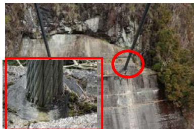
Anchoring to the anchor frame
