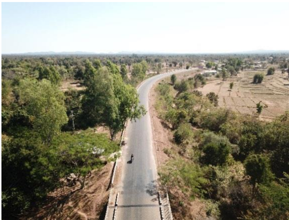
Figure3. 7 The top view of Entrance the bridge to Salavan province
