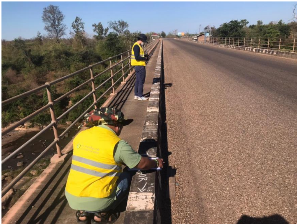
Figure3. 10 General pavement condition of Xebangnouan Bridge
