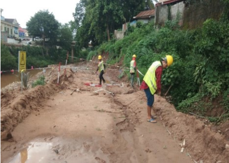
Site barricade at km 0+350 L Thin village
