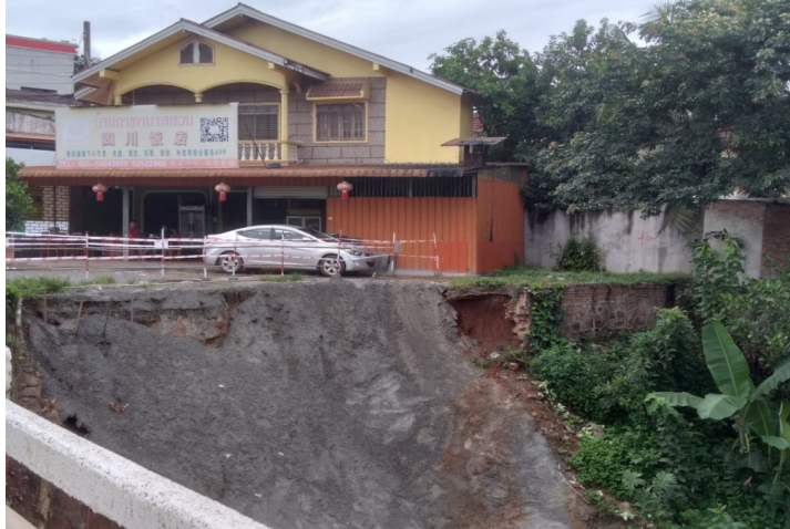
Site barricades (red-and-white vinyl tape) and warning signs at Section R4 station 4+130 R in Nawan Noy village on March 2023
