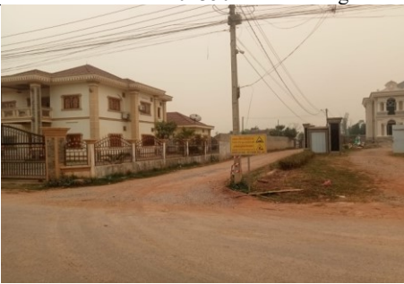
Installation of safety and speed control signs at 2+850 R in Nawhannoy village
