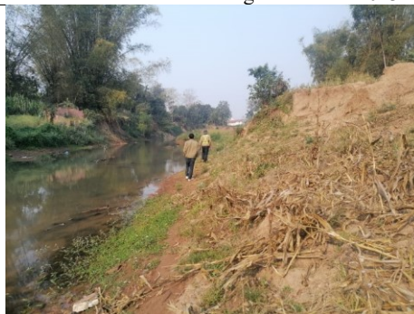
Existing condition at Section L2 in Nalao village on March 2023
