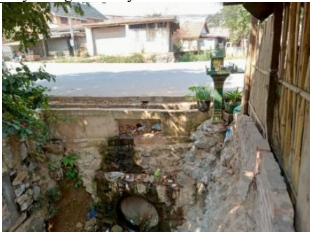
Existing conditions of Drainage/Gate
