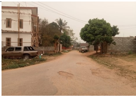
Installation of safety and speed control signs at 4+940 R
