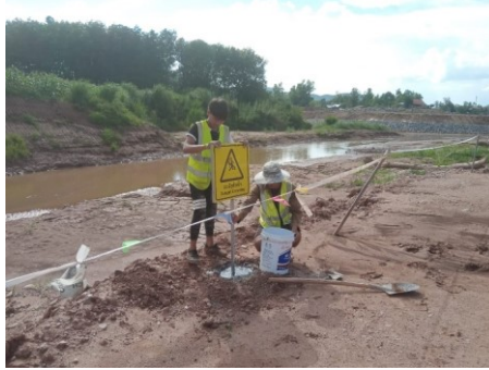
Installation of site barricades (white vinyl tape) in Nawan Noy village
