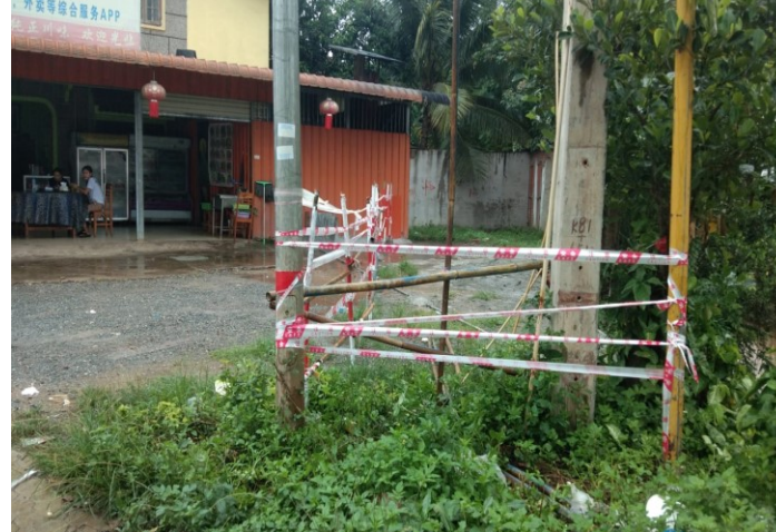
Site barricades (red-and-white vinyl tape) and warning signs at Section R4 station 4+130 R in Nawan Noy village on March 2023
