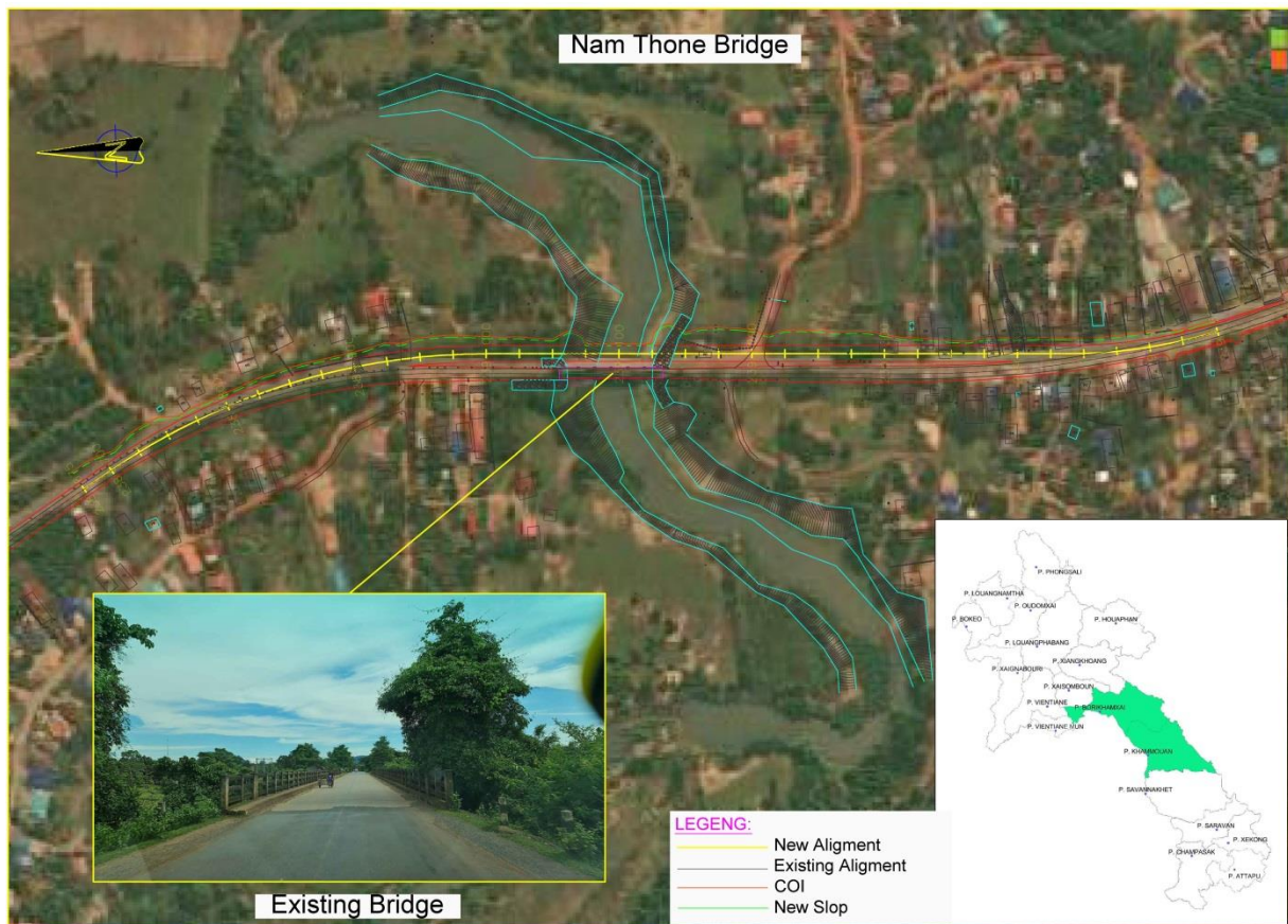
Figure 1-5: Existing Nam Thone Bridge
